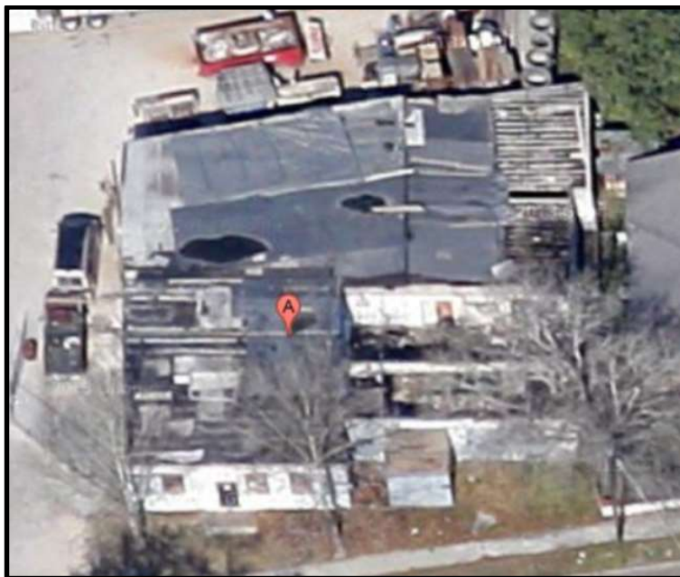
Figure 5. Collapsing roof conditions at the Duval Plating building
