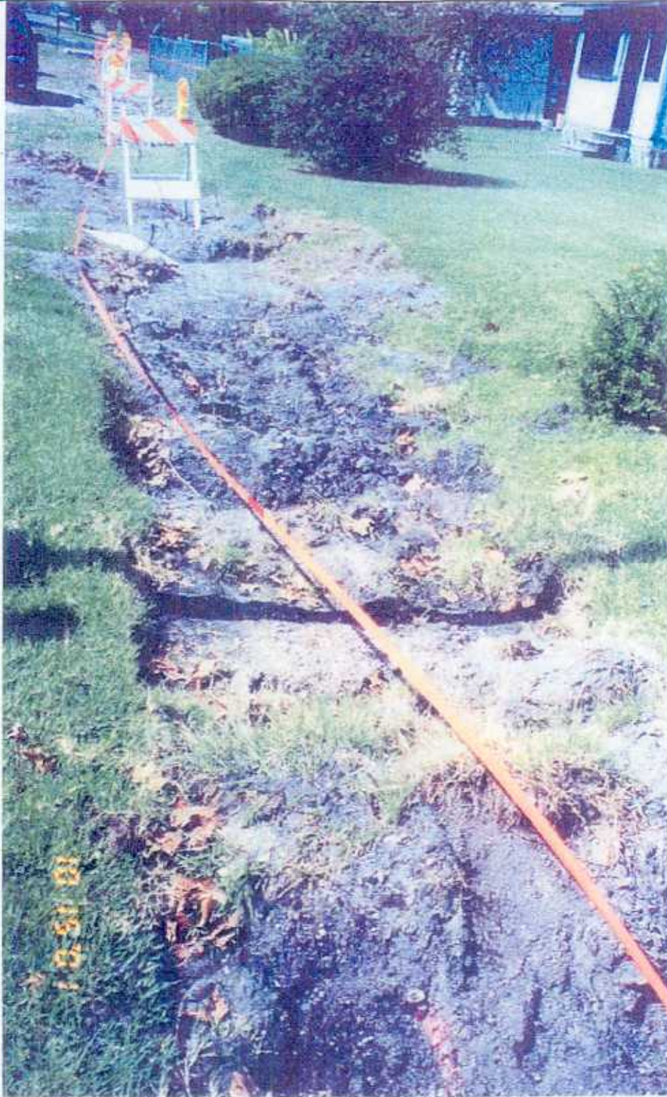
Photograph 12: Mill View neighborhood, sidewalk was replaced due to cracking. This is what the fill looks like without vegetation covering it.
