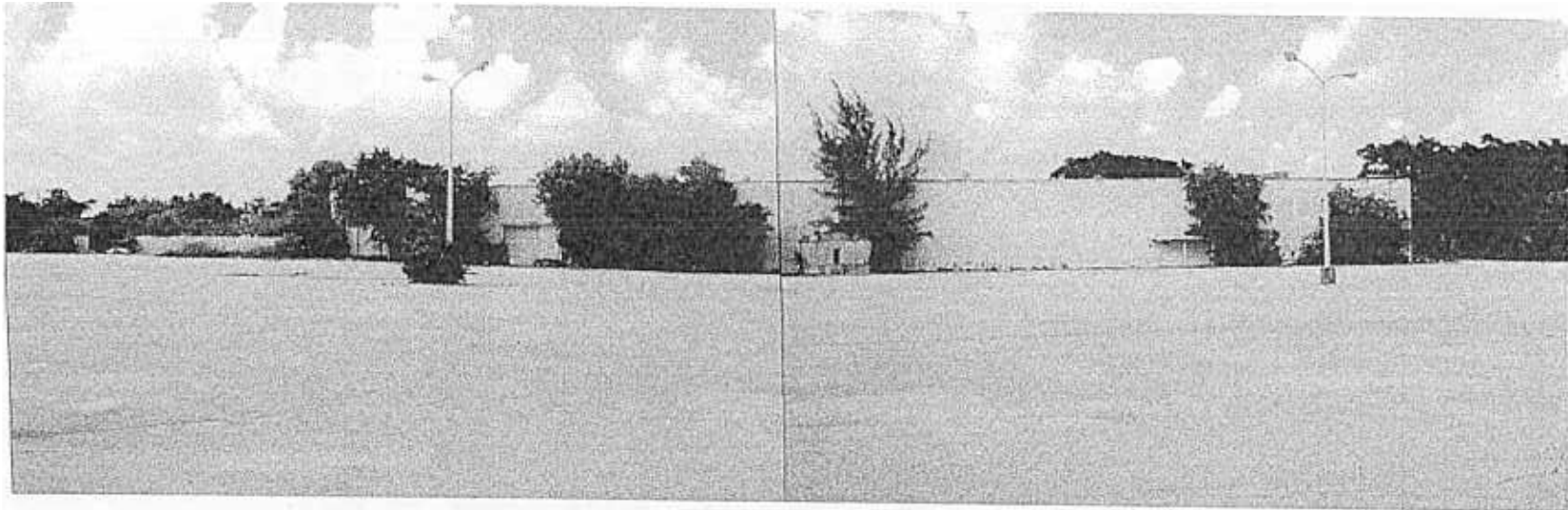
Photo 3: Looking north from the middle of the site, at the south side of the northern building
