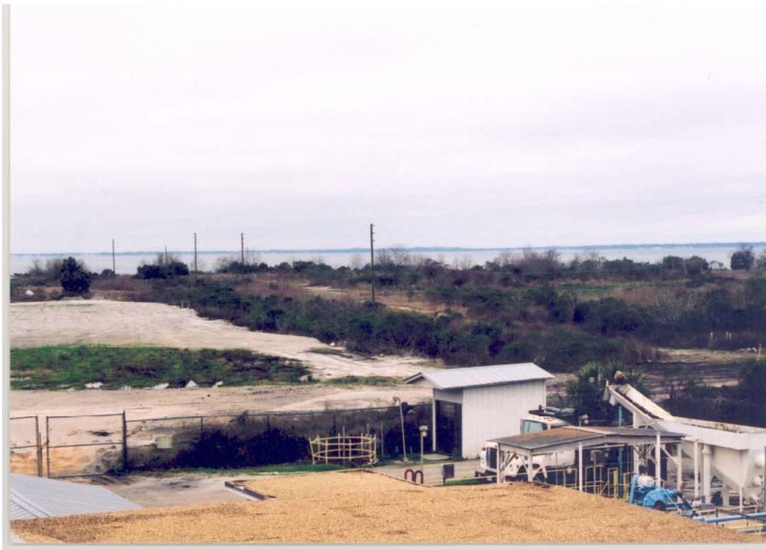
Photo 9: View to the northwest from the bridge, vegetated area forms the southern boundary with the northern part of the site.
