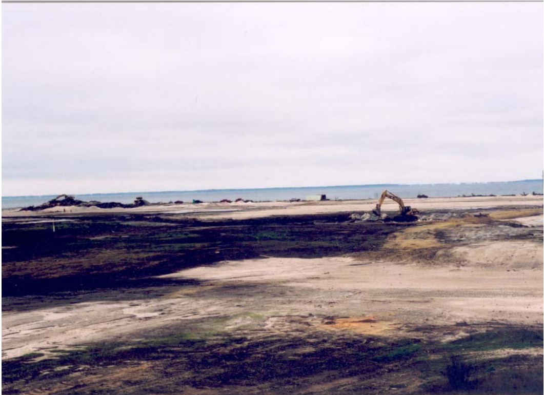
Photo 7: Soil capping operations on the southern parcel.
