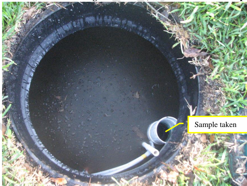
Figure 7 First chamber of Stage 2 biofilter (B-HS2-LIGNO-0" sample)
