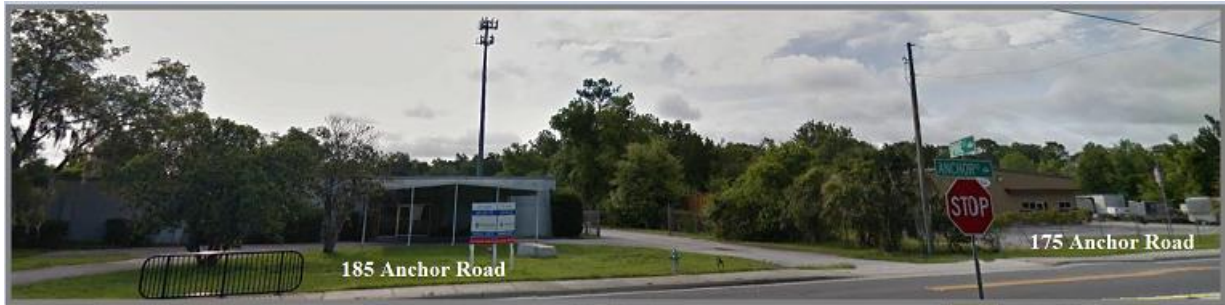
Figure 1: The Anchor Road Solvent Site from Pine Street looking east
