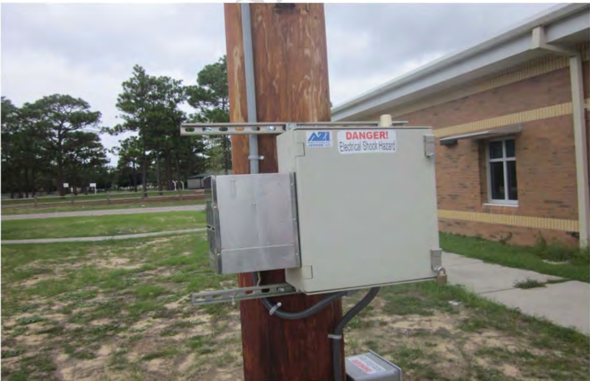
Photo 2. Continuous Hydrogen Sulfide Monitoring Equipment at the Community Center
