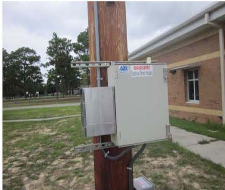
Hydrogen sulfide monitor near the landfill at the Wedgewood Community Center
