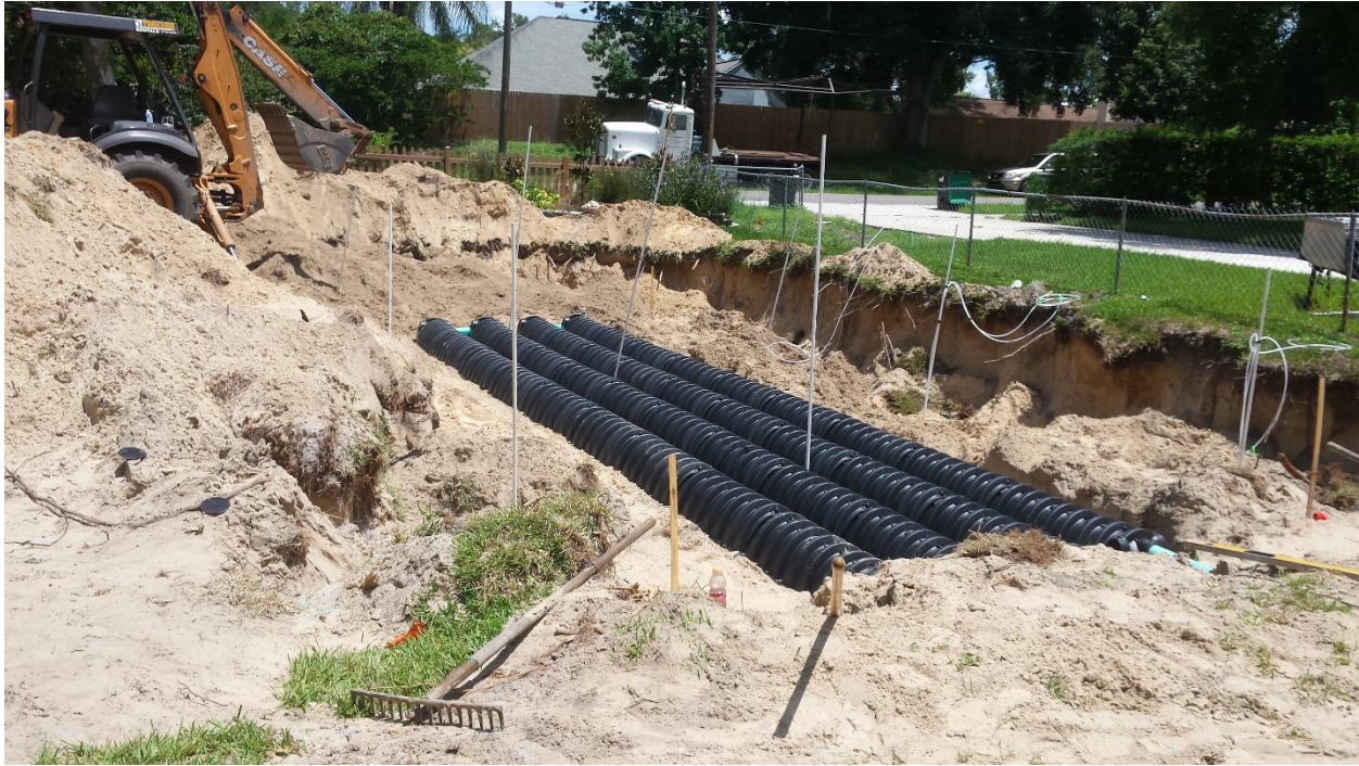
Completed drainfield, piezometers between second and third rows. PVC pipes on edges mark edge of liner. Pipes between infiltrators are piezometers. Tubes go to horizontal wellpoints.
