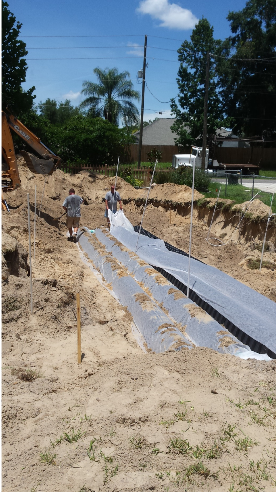
Fabric cover being installed over infiltrators
