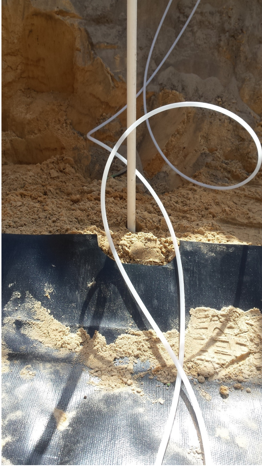
PVC pipe marking location for deep lysimeter, notch in liner to direct flow to lysimeter
