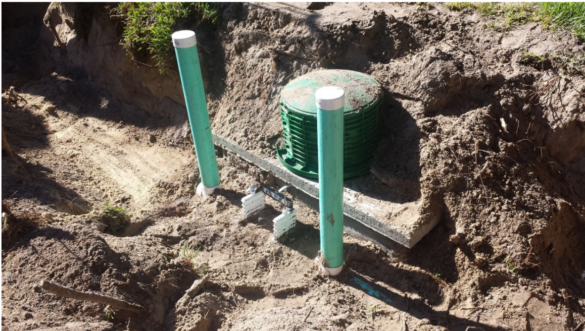
Knife valves and effluent sampling/inspection riser on septic tank. Green pipes are inspection ports to confirm flow direction.
