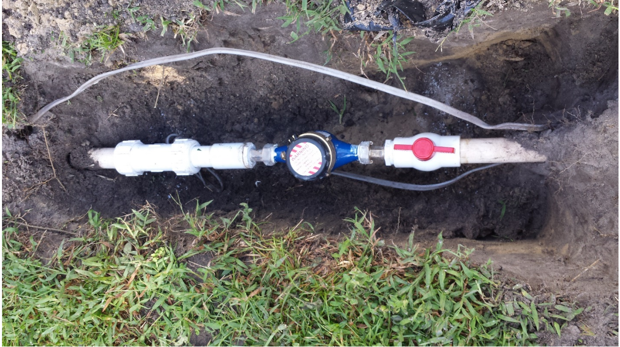
Flow meter installed on supply line to house, next to water well. Irrigation line is separate.
