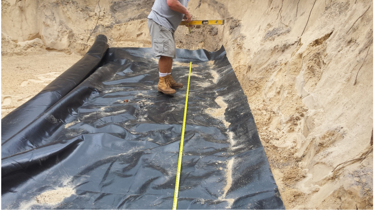
Liner installation, first stage
