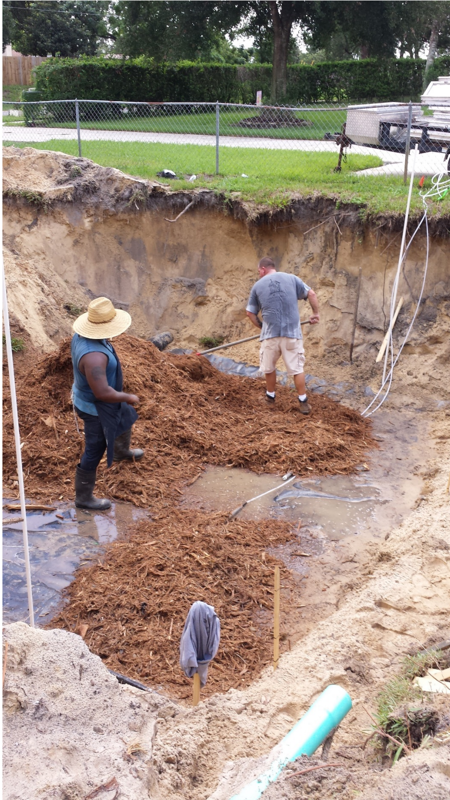
Installing mulch adjacent to compacted sand for header, first stage
