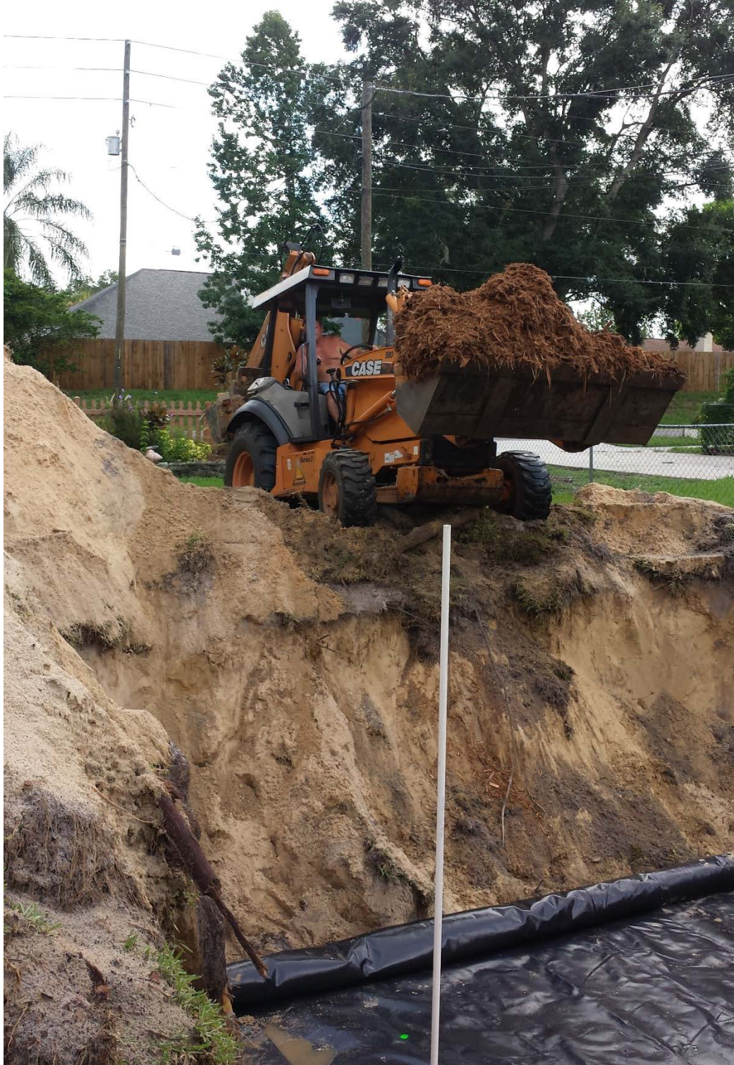
Mulch installation, second stage
