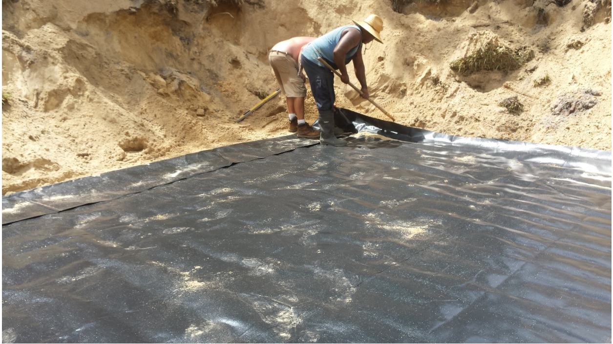
Building up berm around edge of liner
