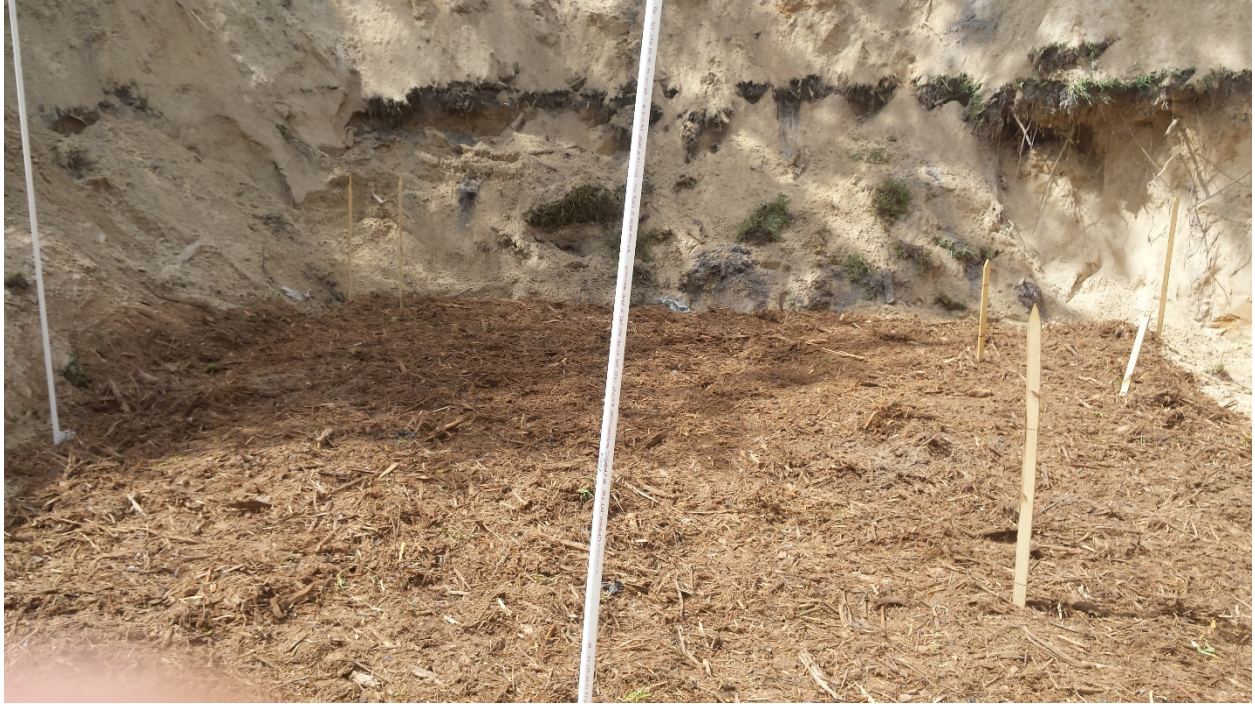
Completed mulch installation. Pipe is piezometer. Stakes used to assure uniform depth of mulch
