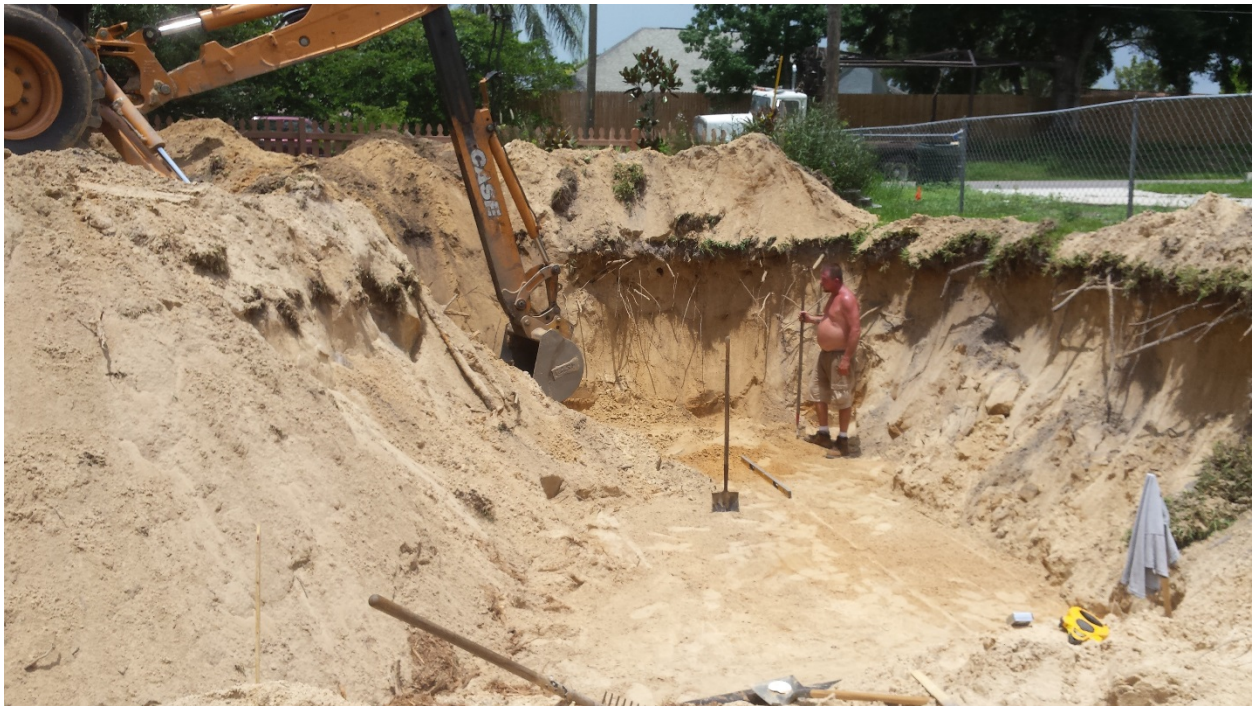
Excavation of pit and leveling for liner installation
