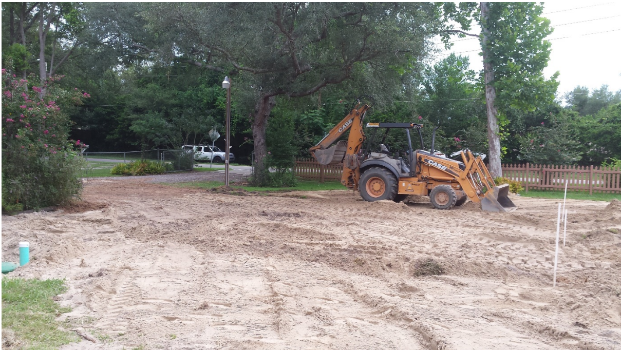
Edge of drainfield and material stockpile and equipment turning area, to be re-sodded
