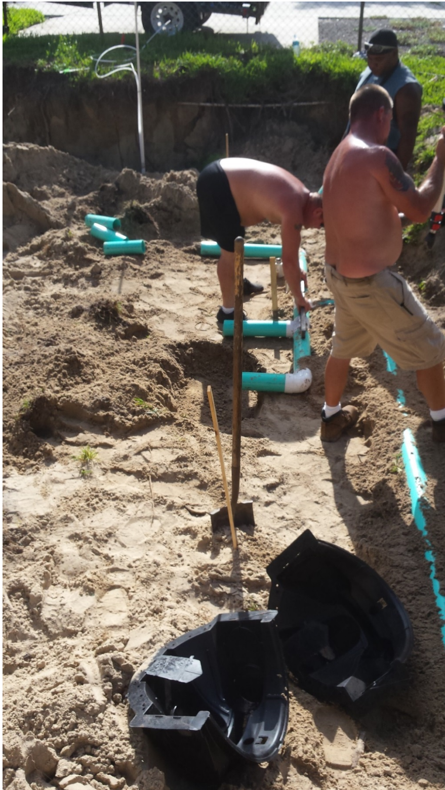
Header installation
