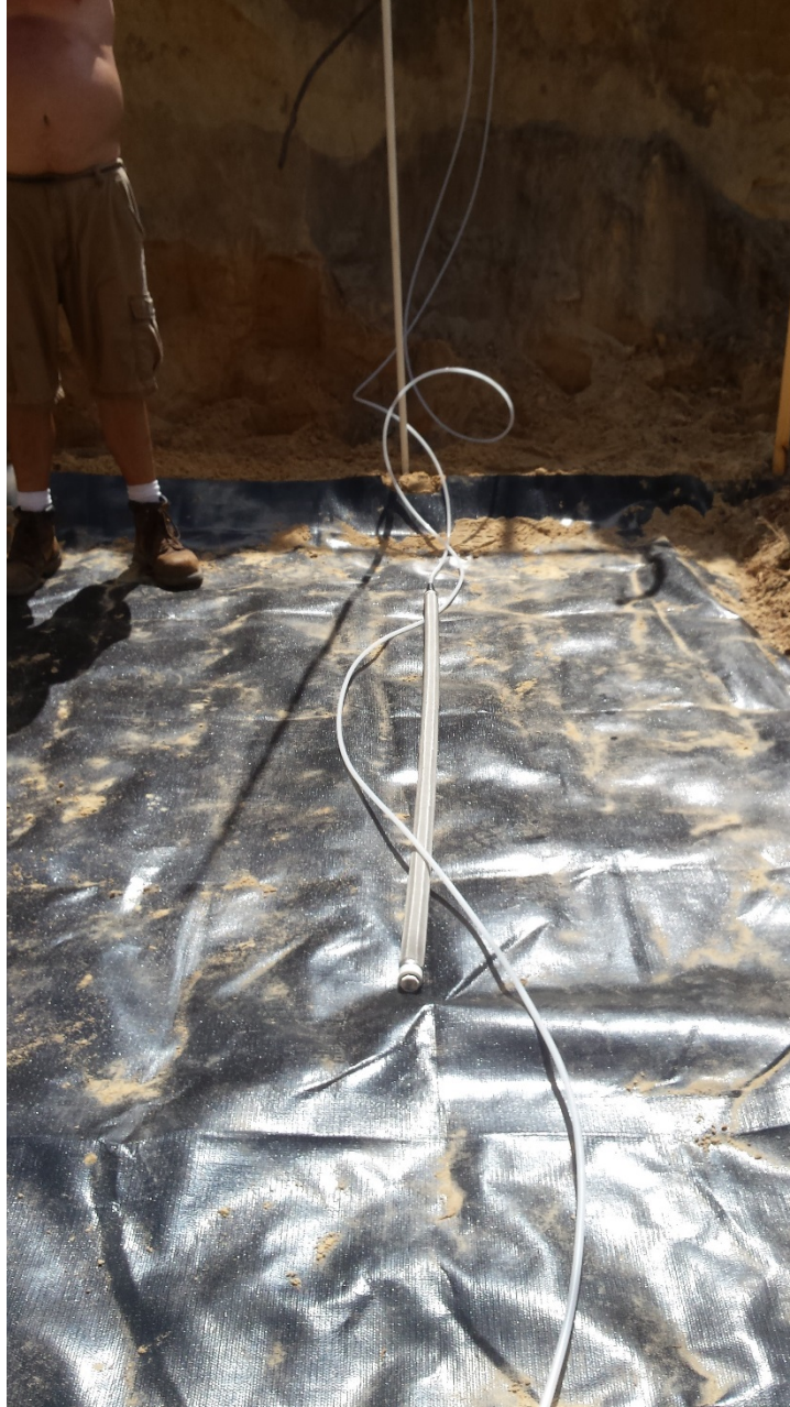
Horizontal wellpoint on liner
