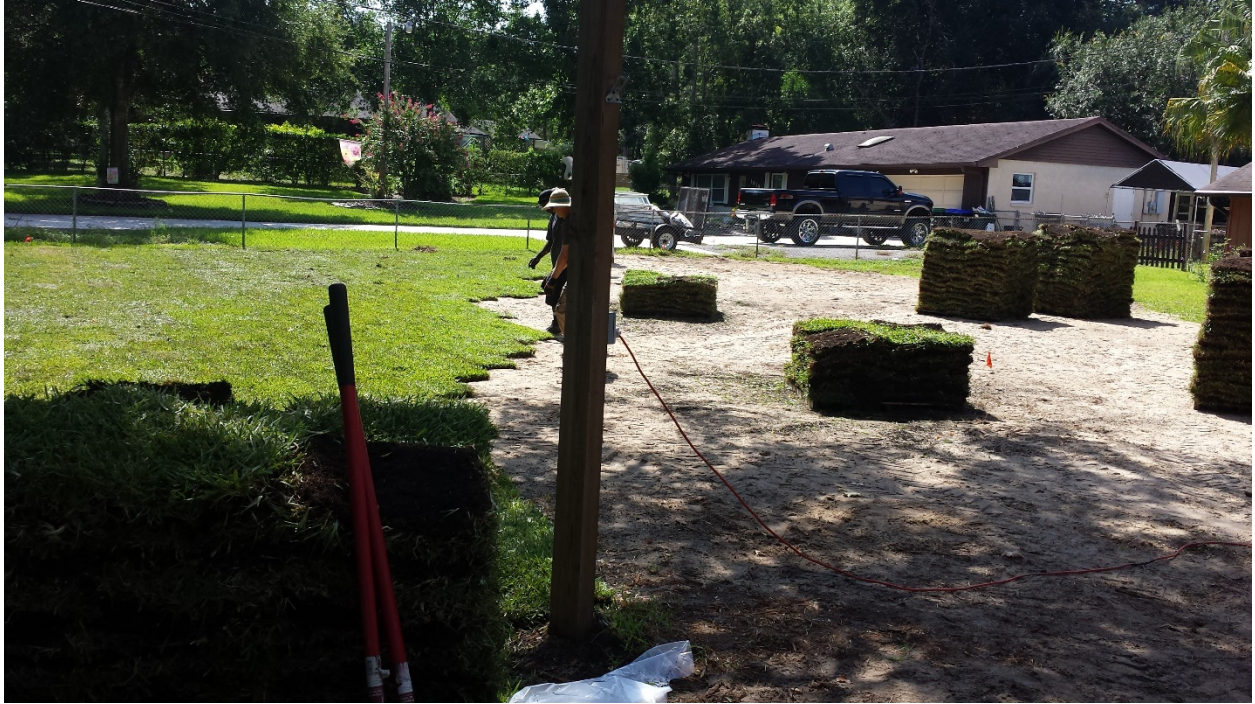
Total of 14 pallets of sod laid to restore damaged area
