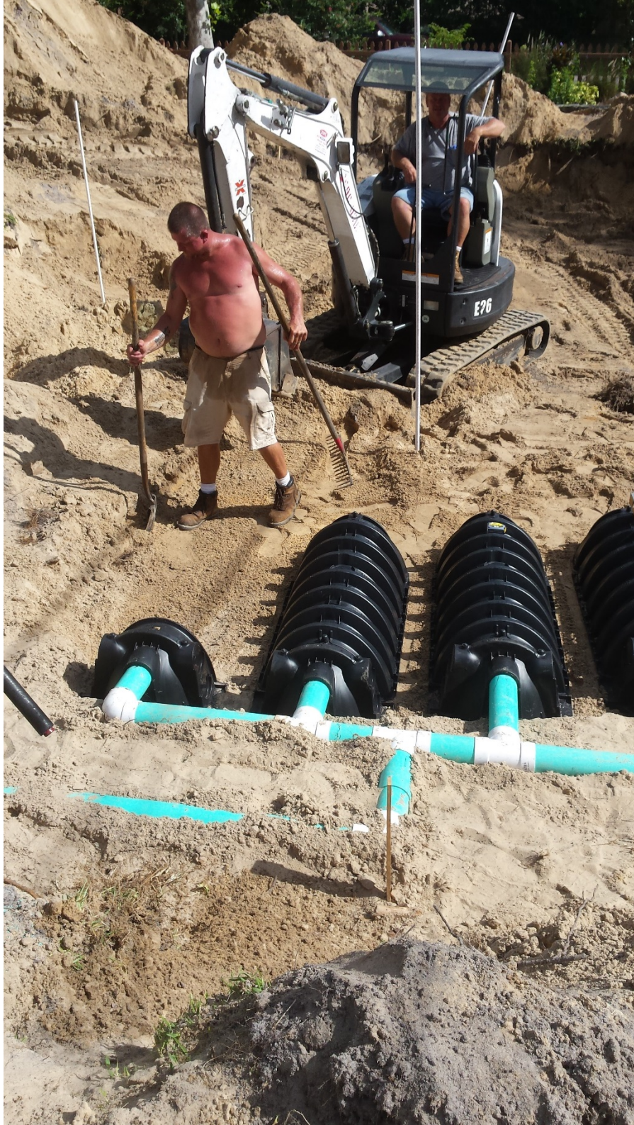
Drainfield installation
