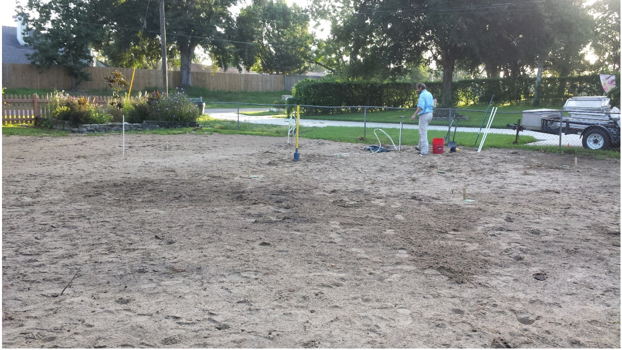
Installing lysimeters in graded drainfield area
