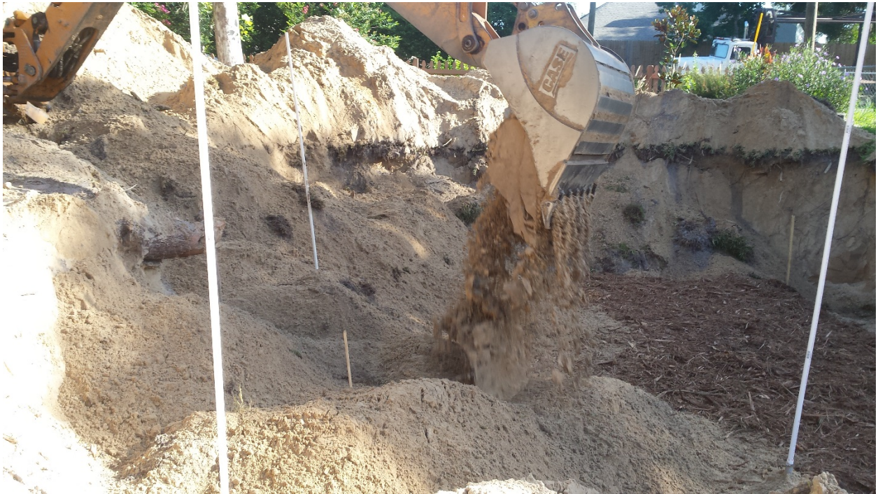
Installing backfill on top of mulch, 19 to 20 inches thick
