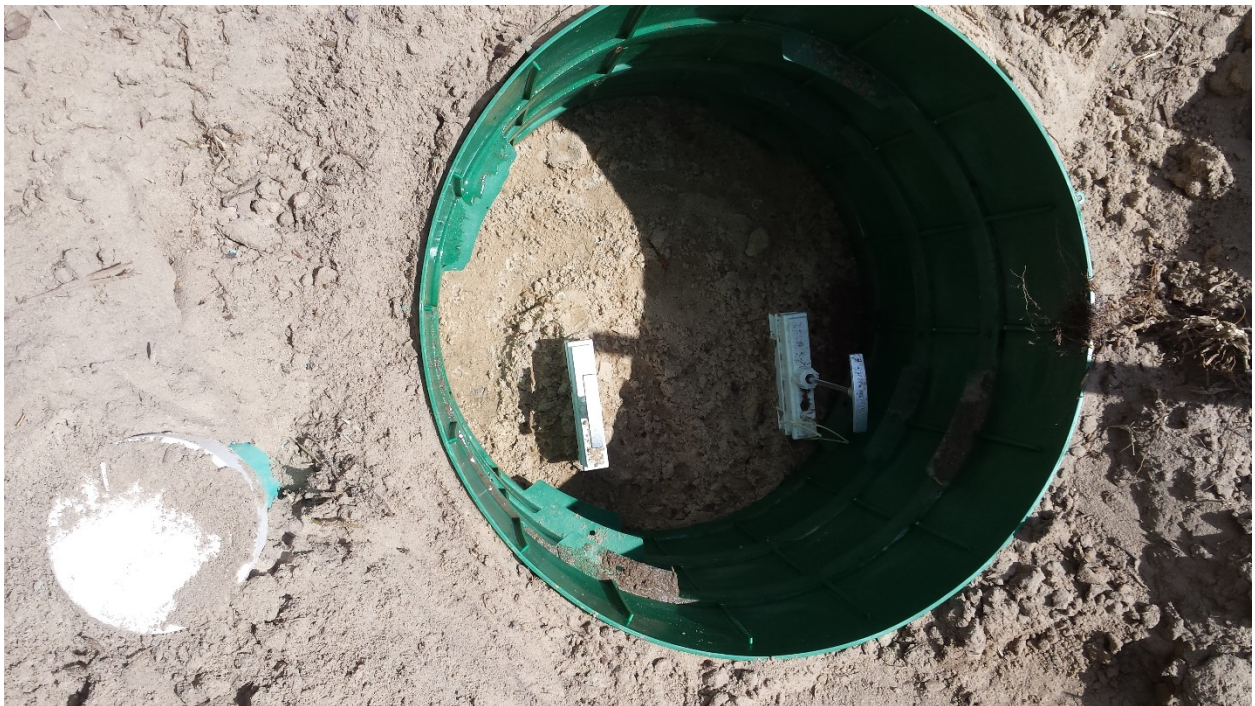
Valve to experimental drainfield opened after flow meter installed
