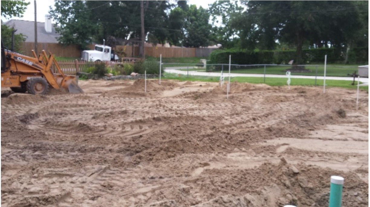
Excavation filled prior to final grading
