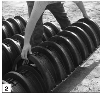
2 Connect the chambers.
