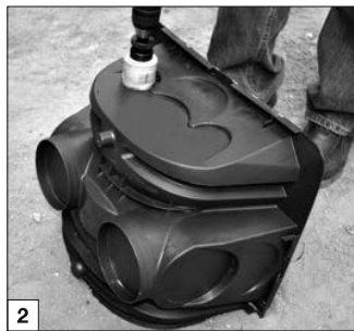
2 Drill pressure pipe hole.
