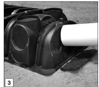
3 Insert inlet pipe.
