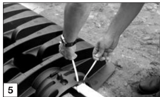
5 Secure pressure pipe.
