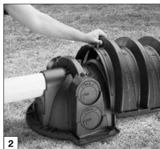
2 Place first chamber onto endcap.
