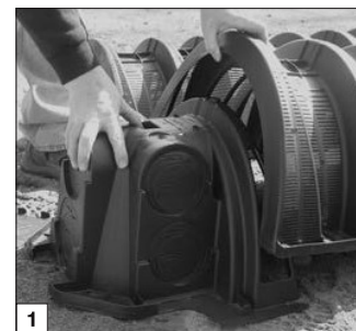
1 Slide endcap under chamber.
