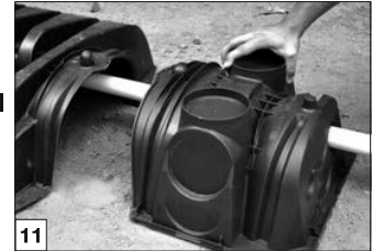
11 Lateral pipe through endcap.
