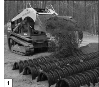
Ladle soil on chamber domes.
