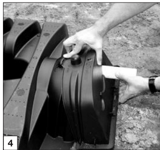
4 Place endcap over inlet end.
