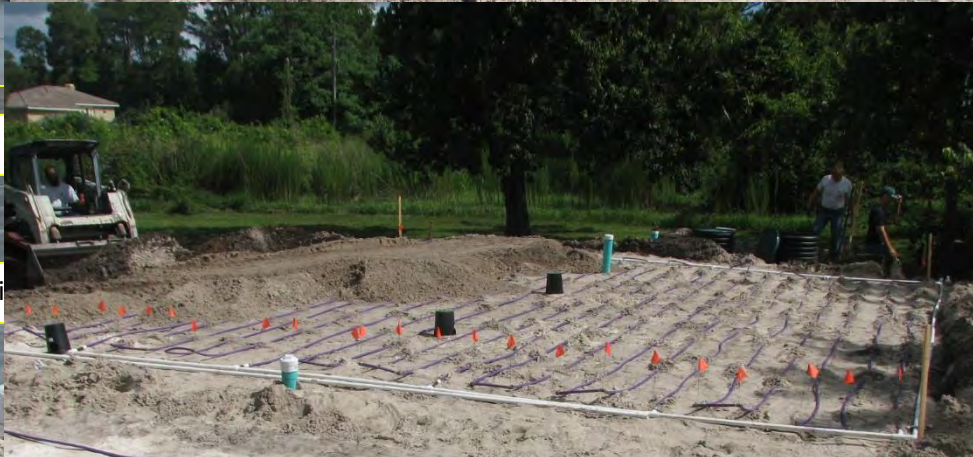
Gravel Underdrain
