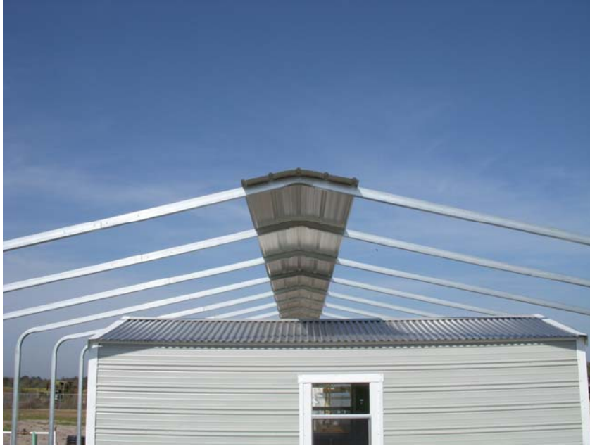
First Roof Panel Installed
