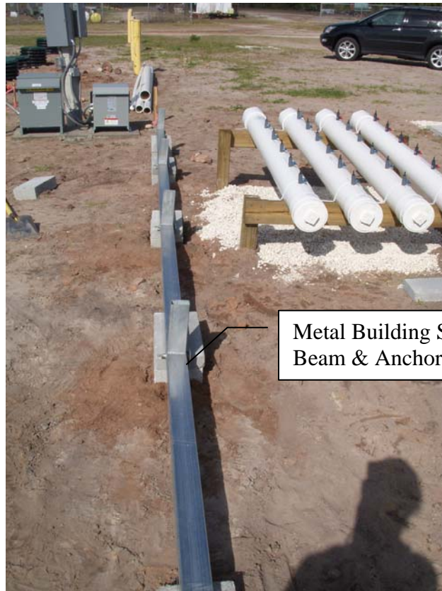
Metal Building Support Beam & Anchors Installed
