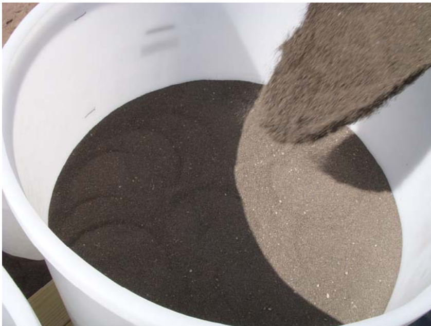
Installing Media in Tank (UNSAT-EC-3) above Geotextile Fabric
