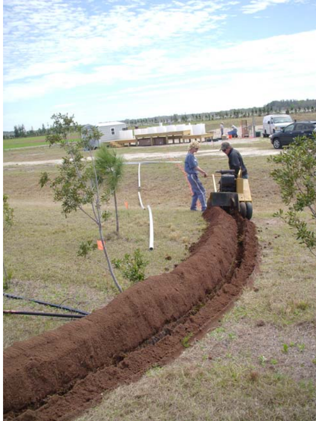
Installing Potable Water Line
