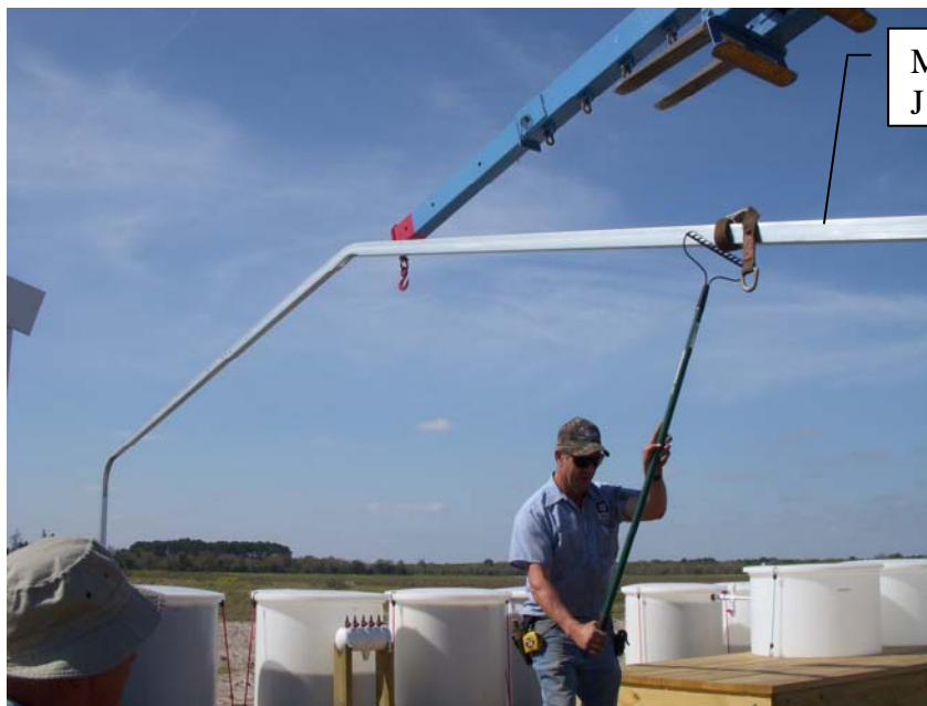
Metal Building J Frame Installed
