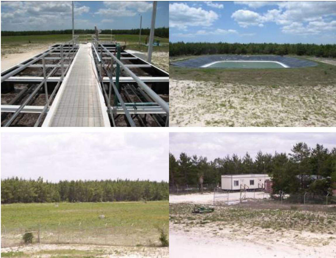
Figure 37. Photos from the Taylor Coastal Centralized Wastewater System Phase 1 Wastewater Treatment Facility (May 24, 2007) showing the package activated sludge plant (top left), holding pond (top right), spray field disposal system (bottom left), and office/workshop (bottom right).
