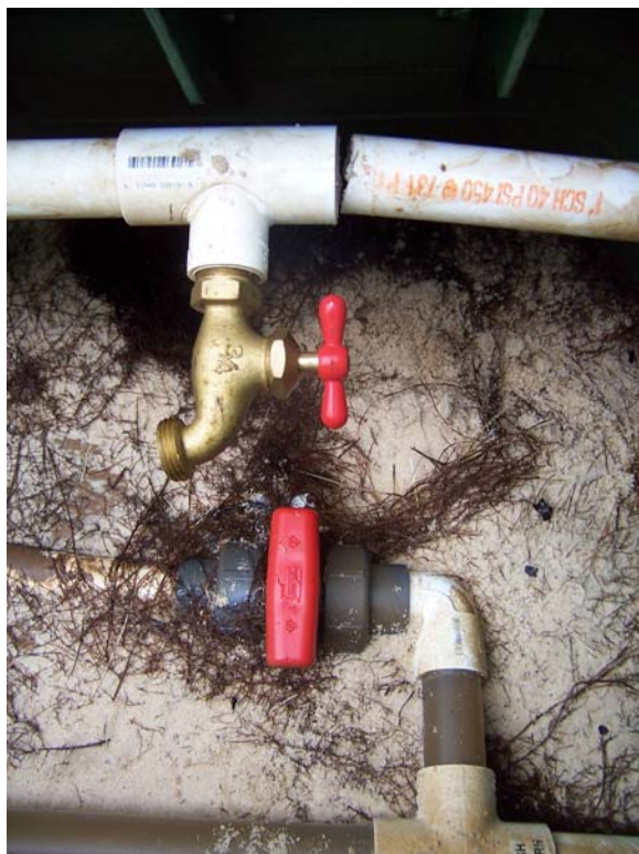
Figure 17. Pictures of site WS-4 taken on April 14, 2009. The broken plumbing evident in this picture was also reported in September 2008. The broken pipe caused the effluent to fill the control box instead of going to the drainfield.
