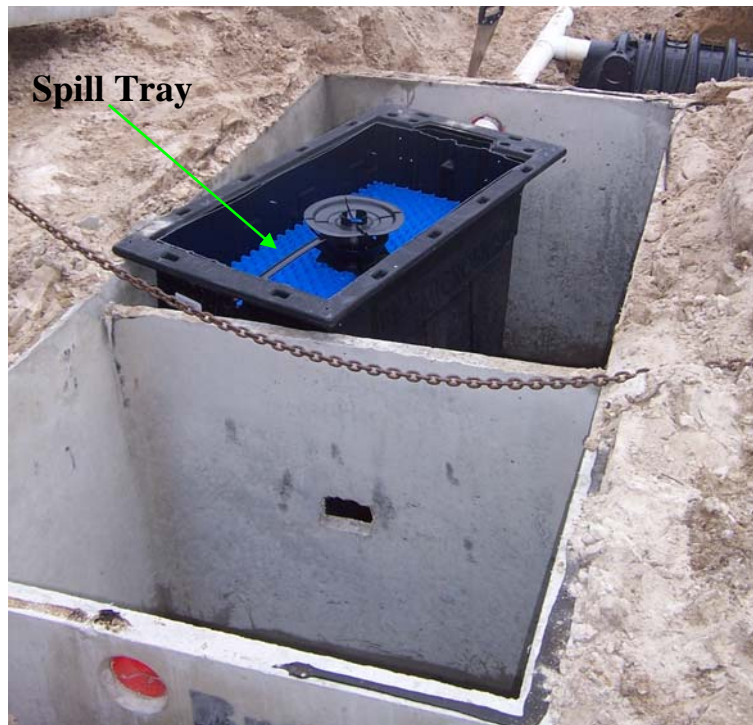
Figure 4. A picture of FAST treatment unit being installed into the treatment chamber of a dual chambered tank. The blue fixed media and spill tray are shown.
