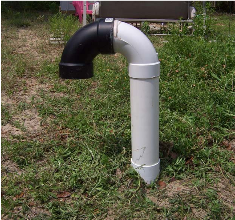
Figure 16. Picture taken on 04/14/09 of a vent pipe typical of FAST installations. Note the PVC coupling at ground level. In order to take a sample, the pipe was cut and repaired with the coupling. The black piece is a charcoal filter installed due to odor complaints. In this neighborhood, there are 5 systems in a row, backing to another 5 systems. This resulted in 10 systems on 1 ¼ acre which apparently created an odor problem.
