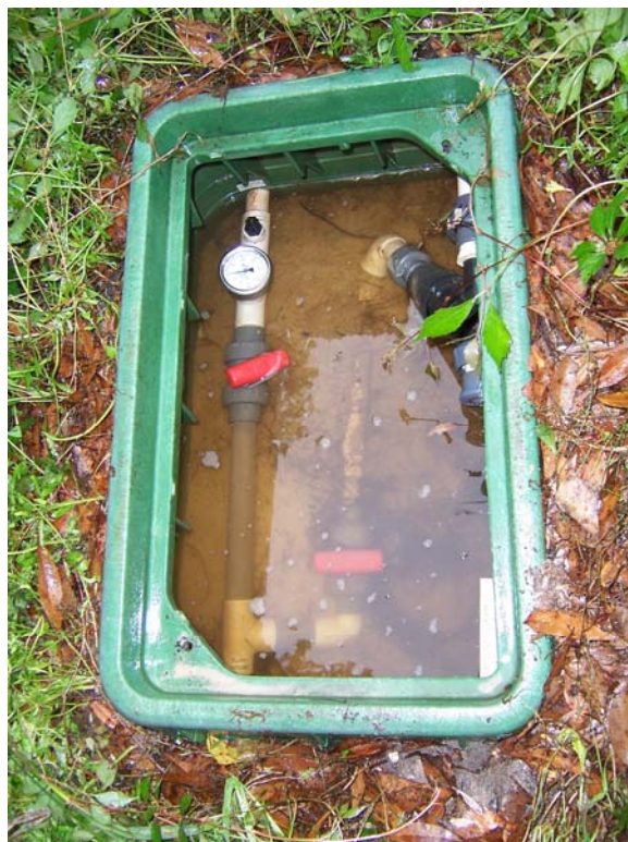
Figure 17. Pictures of site WS-4 taken on April 14, 2009. The broken plumbing evident in this picture was also reported in September 2008. The broken pipe caused the effluent to fill the control box instead of going to the drainfield.
