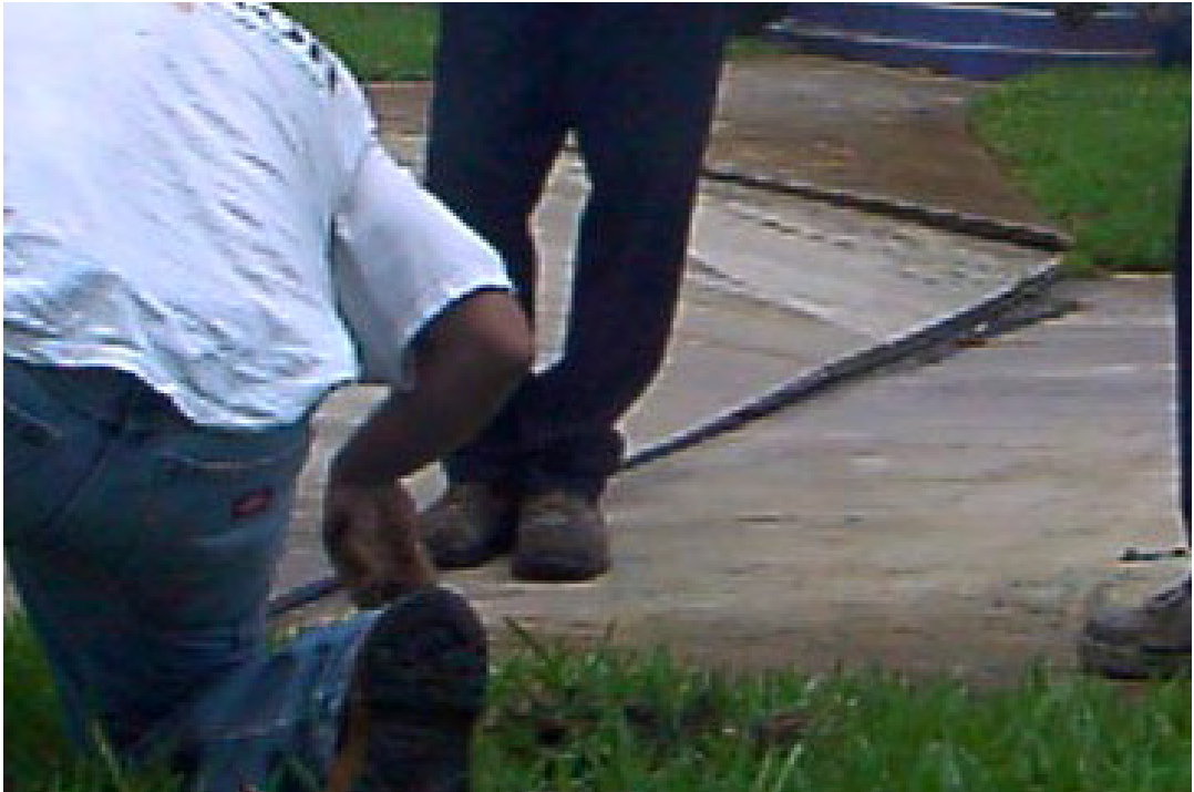
Photo 3: Structural damage due to subsidence in driveway.
