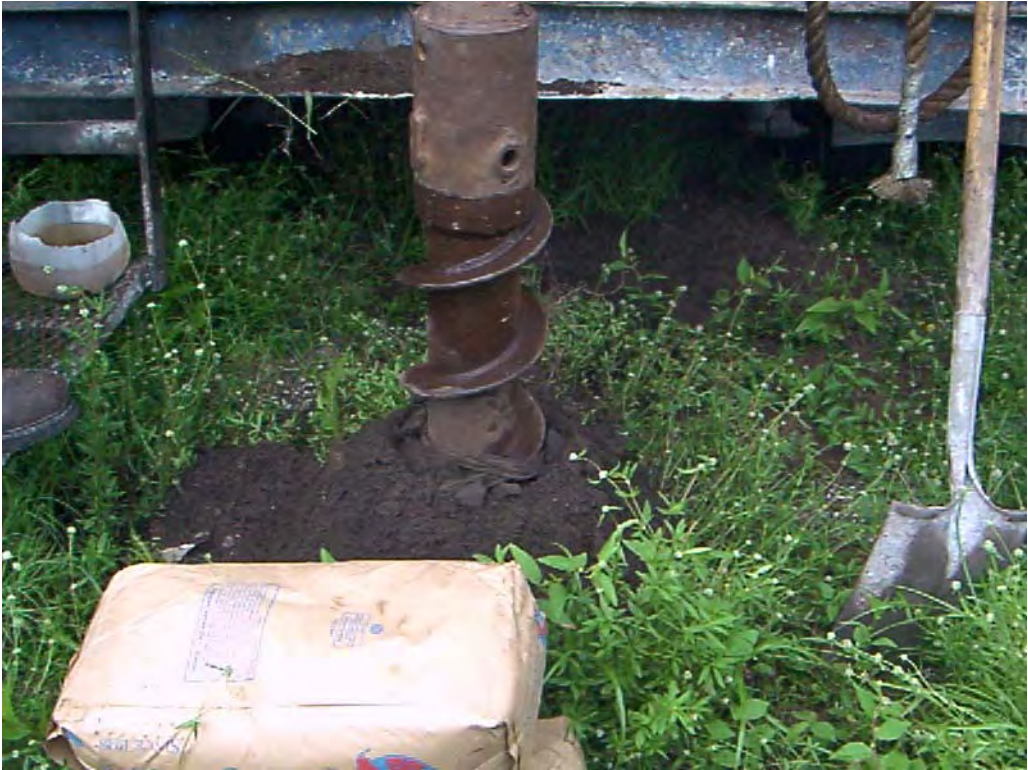
Photo 1: Natural soil DEP's contractors encountered installing a monitoring well.
