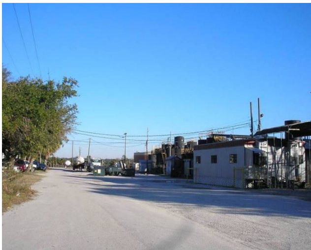
Photo 11 Industrial Water Services looking east on 7 th Street
