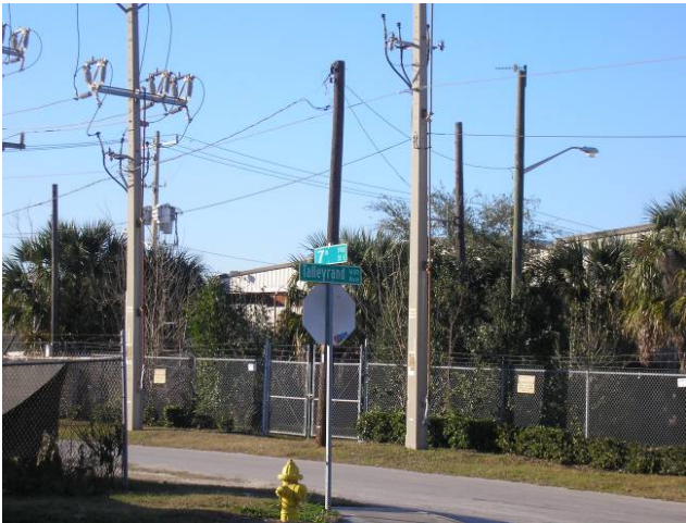
Photo 9 Intersection of 7 th Street and Talleyrand Avenue
