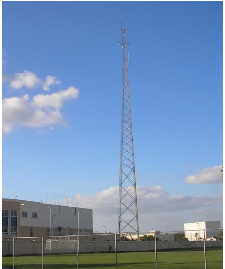
Radio tower, used for communication between field units and the base station
