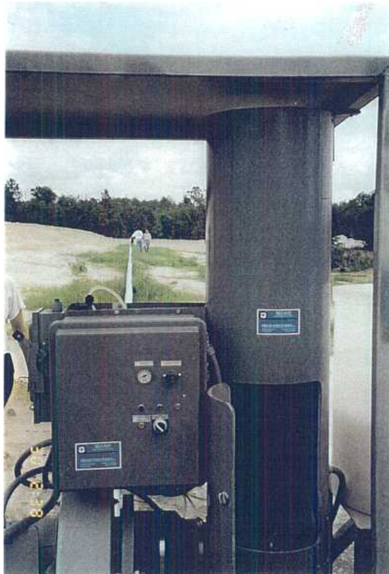
Photograph 10. Closeup of the mister control panel on the south side of the operational C & D cell.
