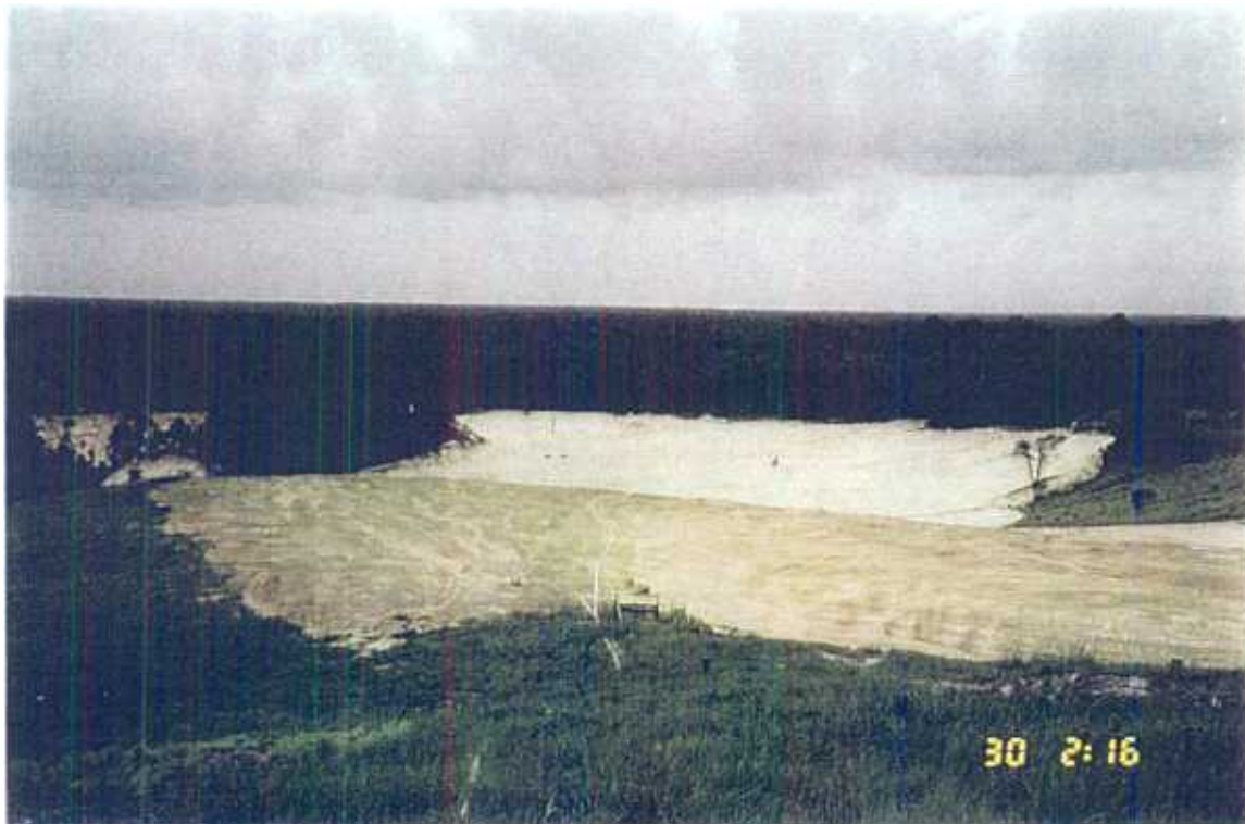
Photograph 4. View to the northwest from the northwest edge of the closed C & D cell
