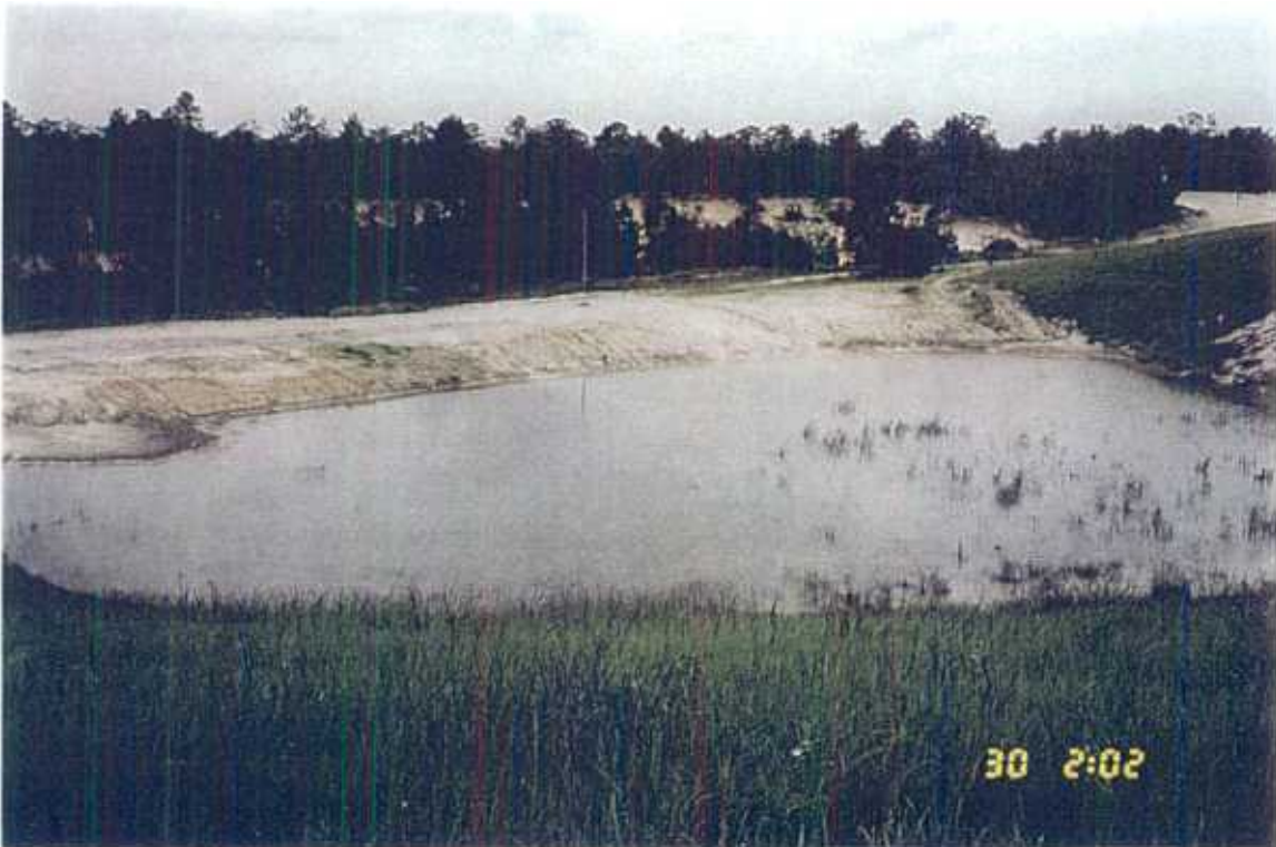
Photograph 2. View to the northwest from the southwest edge of the closed C & D cell.
