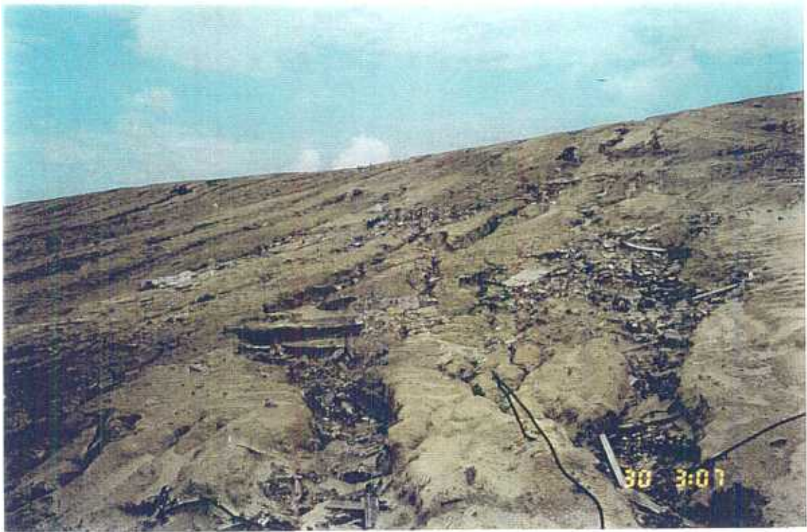
Photograph 9. Erosion on the west side of the currently operating C & D cell.
