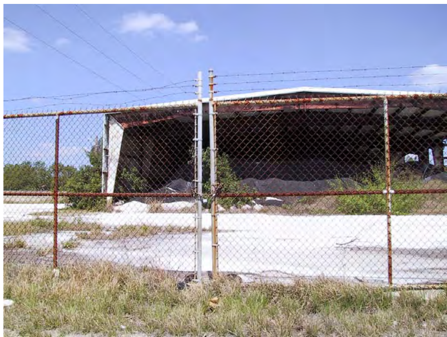
Photo 6. Cover over stored soil at Chloride Metals, Inc.
