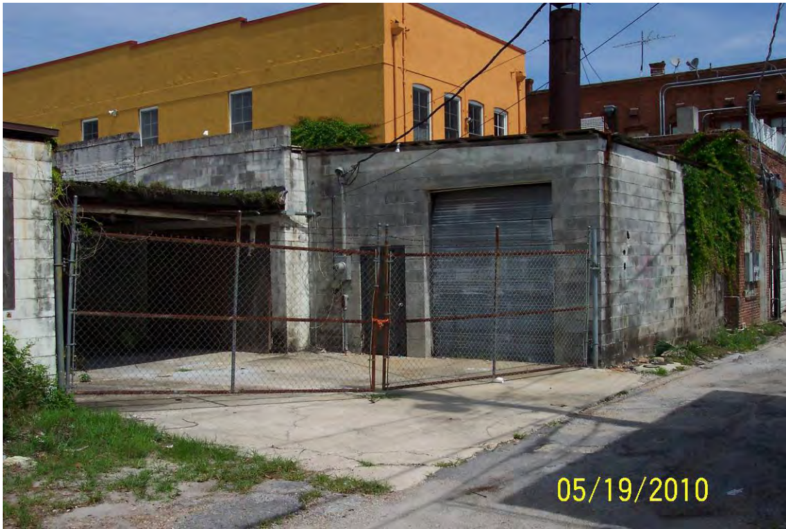
Figure 5. SDC site, view of locked gate at rear of building looking NNW [site visit 051910].
