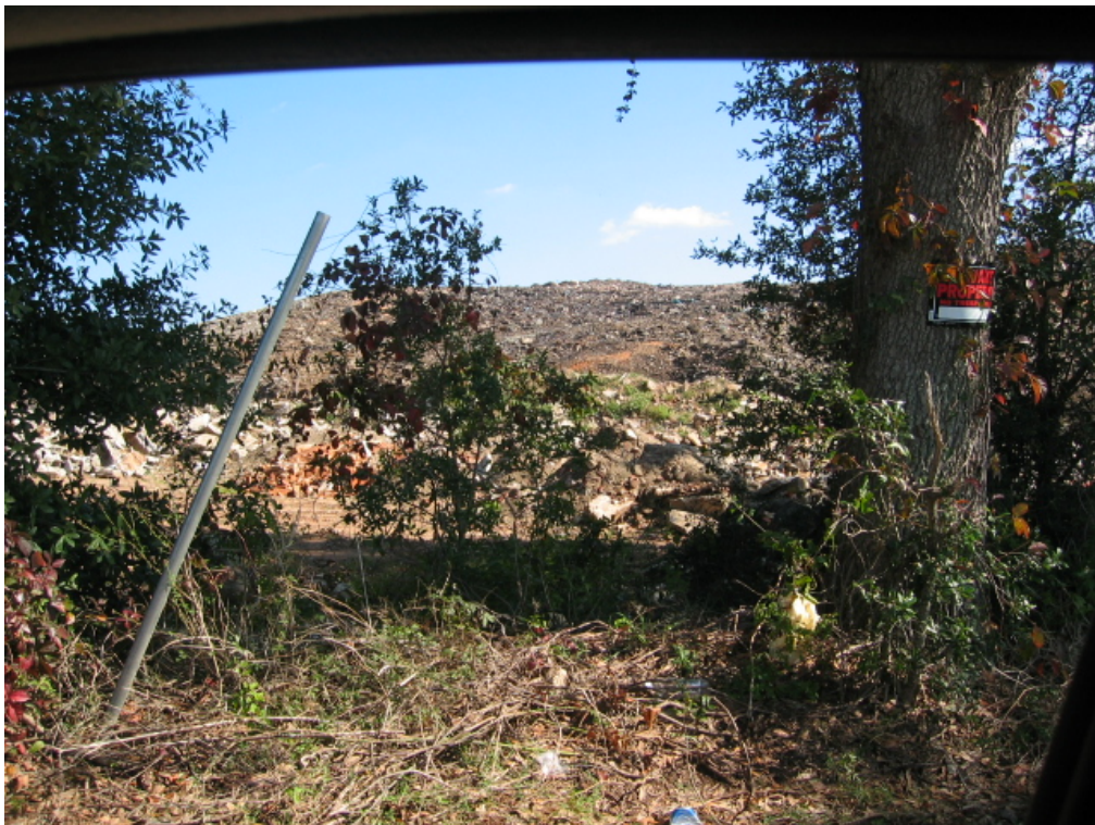
Photo 6: Breach in the chain-link fence west of the site (from East Fence Road).
