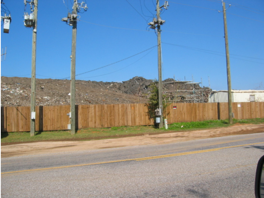
Photo 3: Southeast corner of Saufley Landfill from Saufley Field Road, before covering.
