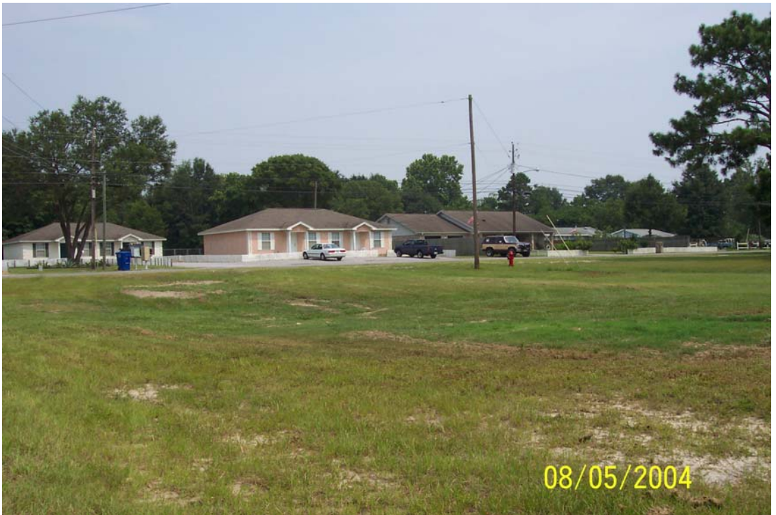
Photo 3: Looking east from Flight Avenue across the utilities corridor to Bob Little Road. Land subsidence is apparent in the center of the photo, homes in background are not part of subdivision.
