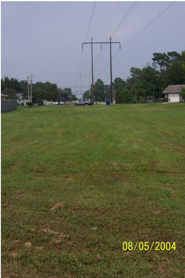
Photo 5: Looking northeast along utilities corridor, land subsidence.
