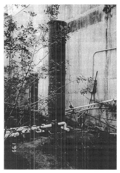
Photograph 9, air stripping tower on the north site of the building, doorframe visible in the background, door has been removed.
