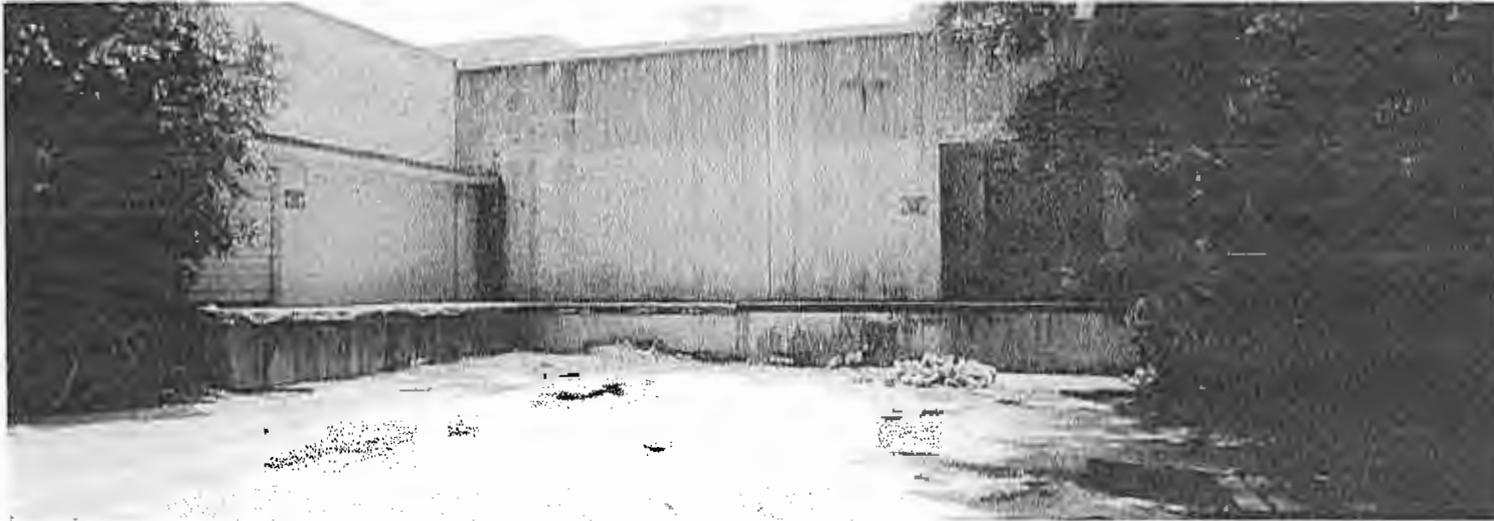
**Photo 6:** Northwest corner of the northern building, shows good condition of the loading dock and profuse vegetation growing on exposed soils.
