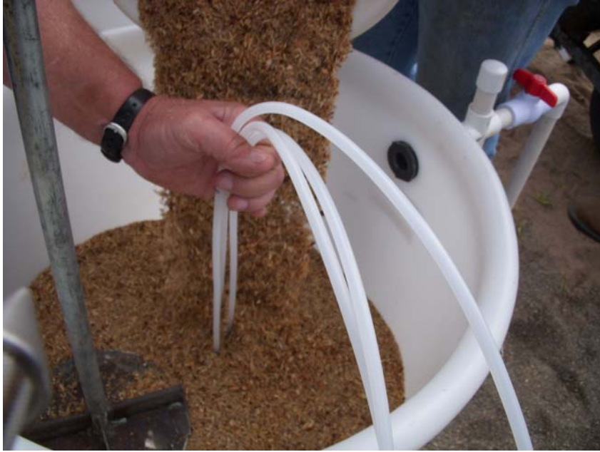
Installing Sample Piezometers within Stage 2 Upflow Tank (DENIT-LS-2)
