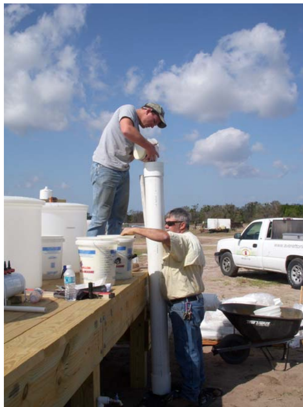
Installing Media within 6" x 72" L Stage 2 Filters (DENIT-SU-1)
