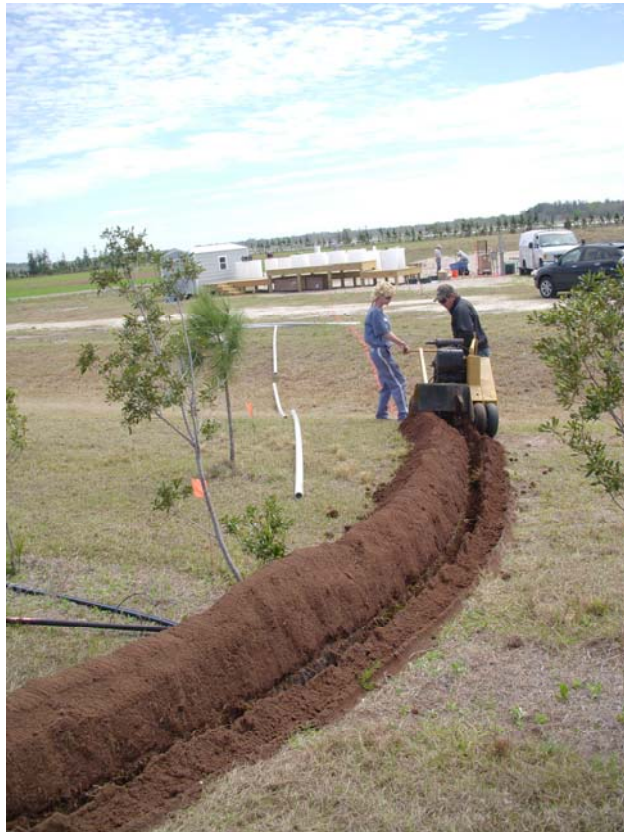
Installing Potable Water Line
