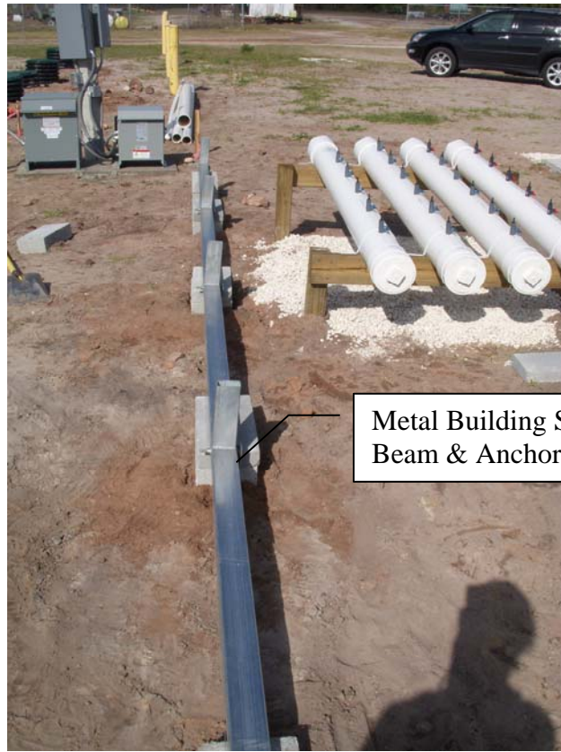
Metal Building Support Beam & Anchors Installed
