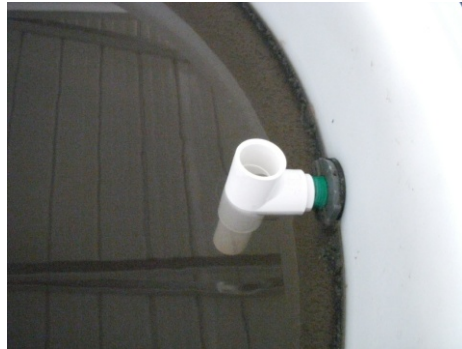
Figure A.6 Outlet Tee in Recirculation Tank
