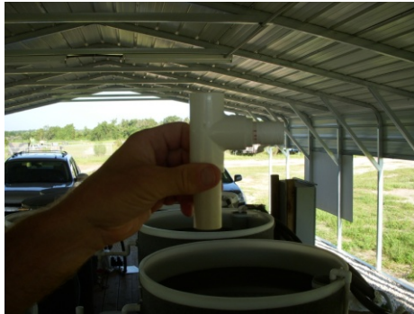
Figure A.6 Outlet Tee in Recirculation Tank
