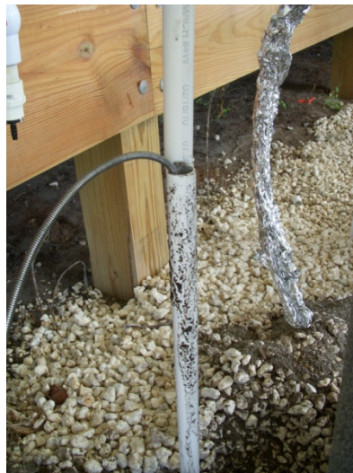
Figure A.7 Unclogging UNSAT-LS4 Influent Pipe
