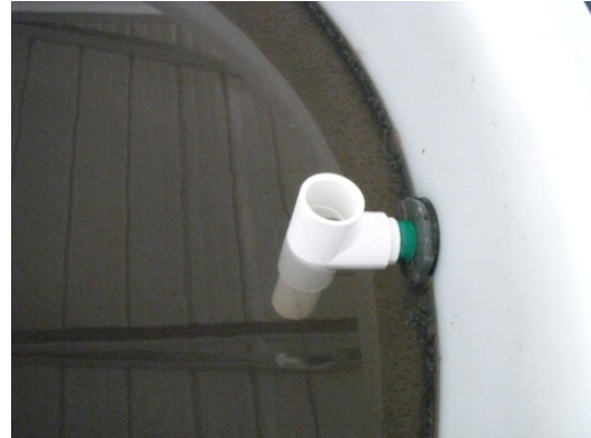
Figure A.3 RC1 Outlet Tee 8/4/10
