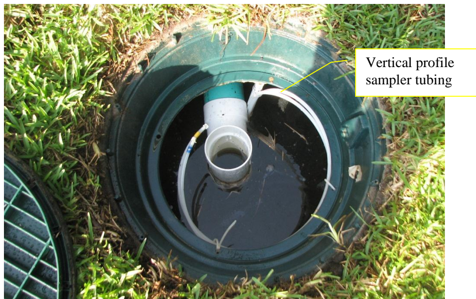
Figure 17 Stage 2 biofilter sulfur chamber
