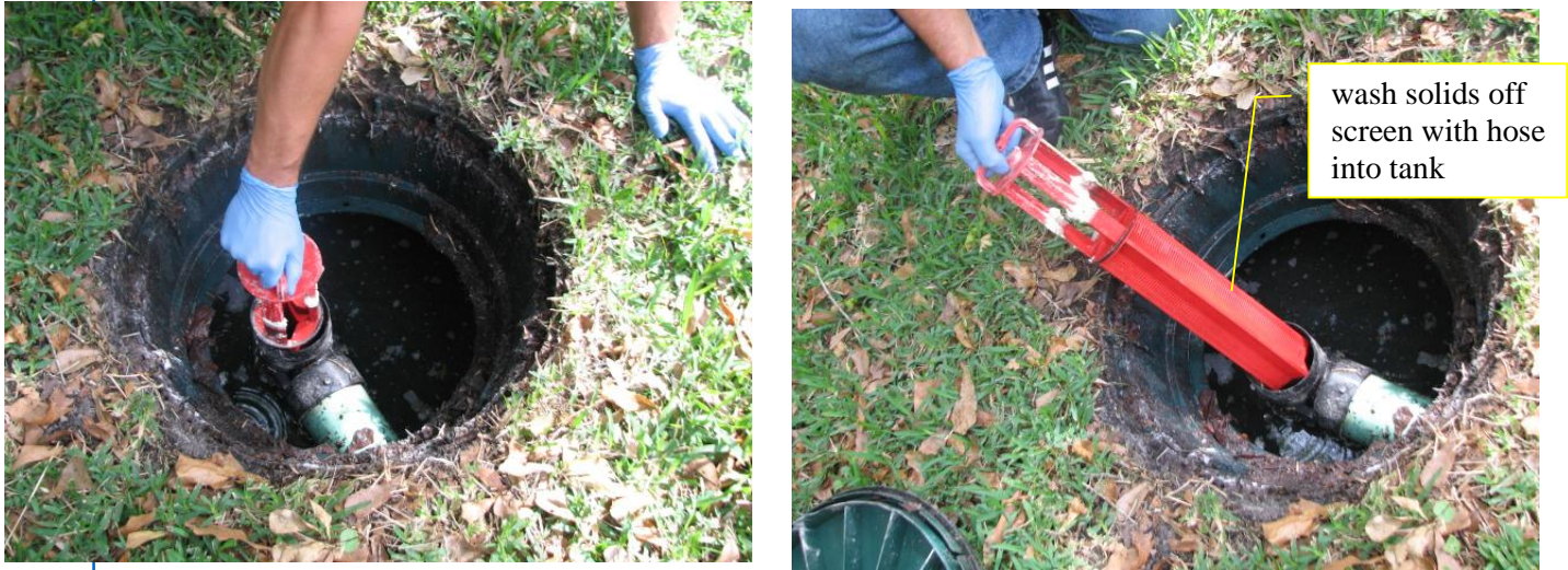
Figure 5 Effluent screen removal
