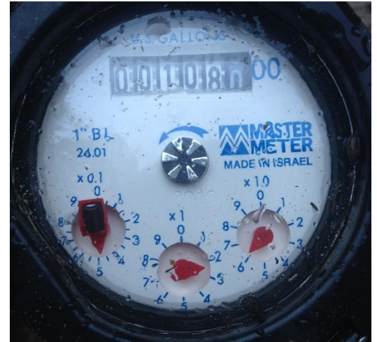
Figure 11 Stage 1 biofilter flowmeter (will not change in single pass mode)
