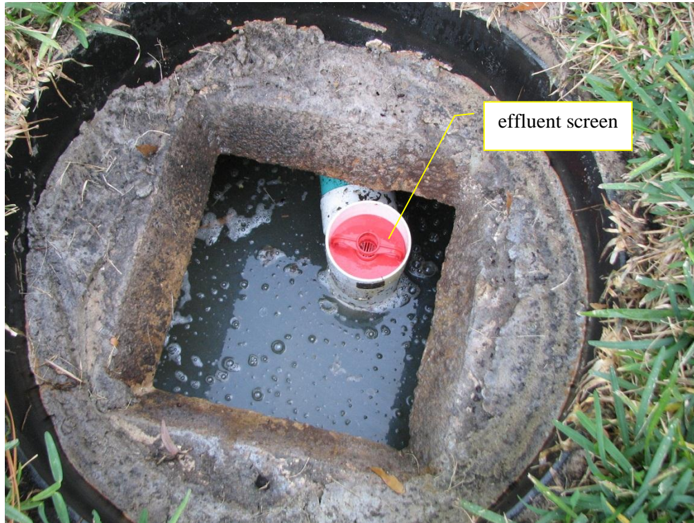
Figure 4 Primary (septic) tank effluent screen
