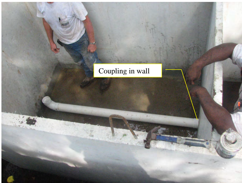
Figure 21 Stage 2 biofilter tank perforated pipe along bottom (lignocellulosic chamber)
