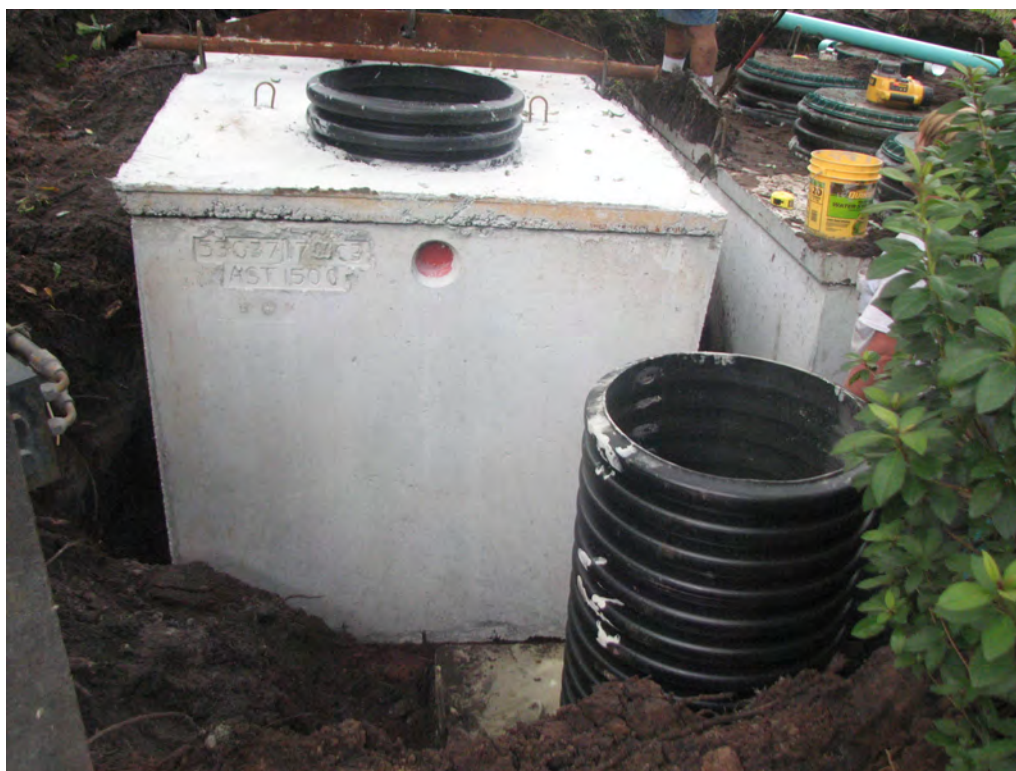
Figure 20 1,500 gallon stage 2 biofilter tank
