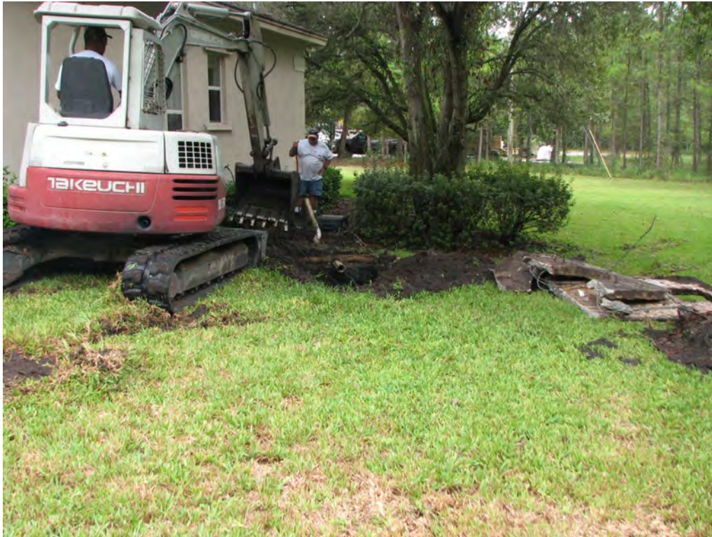
Figure 3 Old septic tank removed
