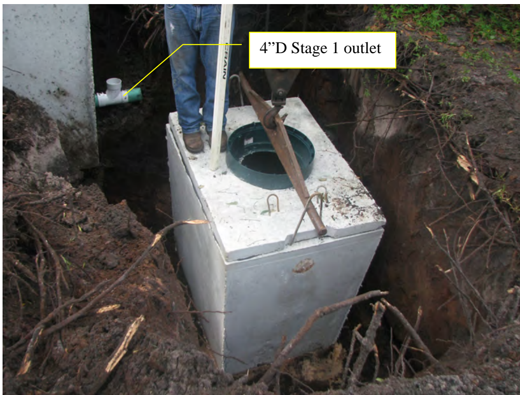
Figure 16 300 gallon pump tank
