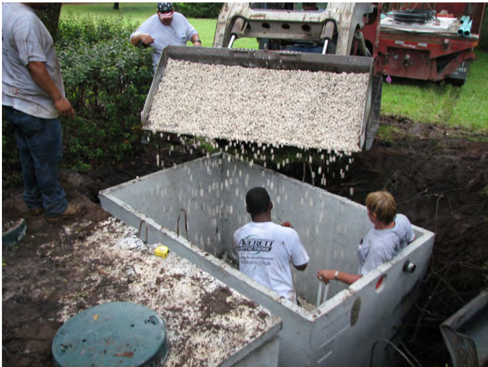
Figure 8 Stage 1 biofilter gravel underdrain
