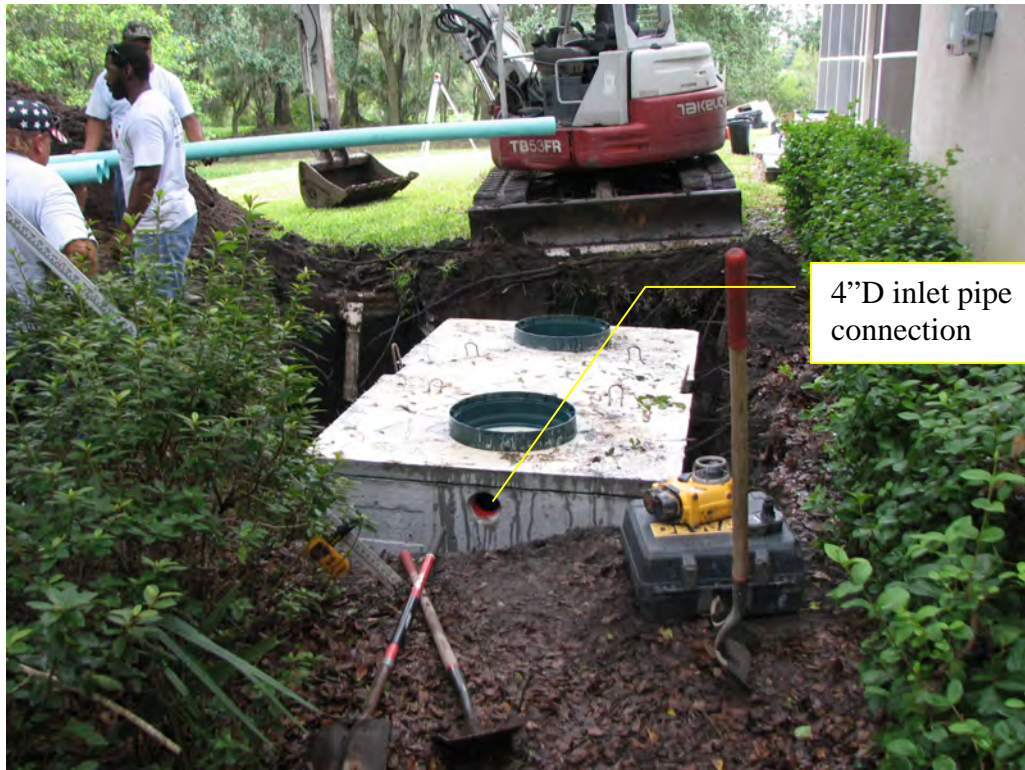
Figure 4 1,050 gallon, two chamber, primary Tank
