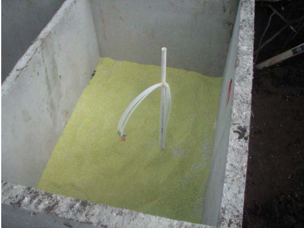
Figure 23 Stage 2 biofilter tank (sulfur mixed with oyster shell)
