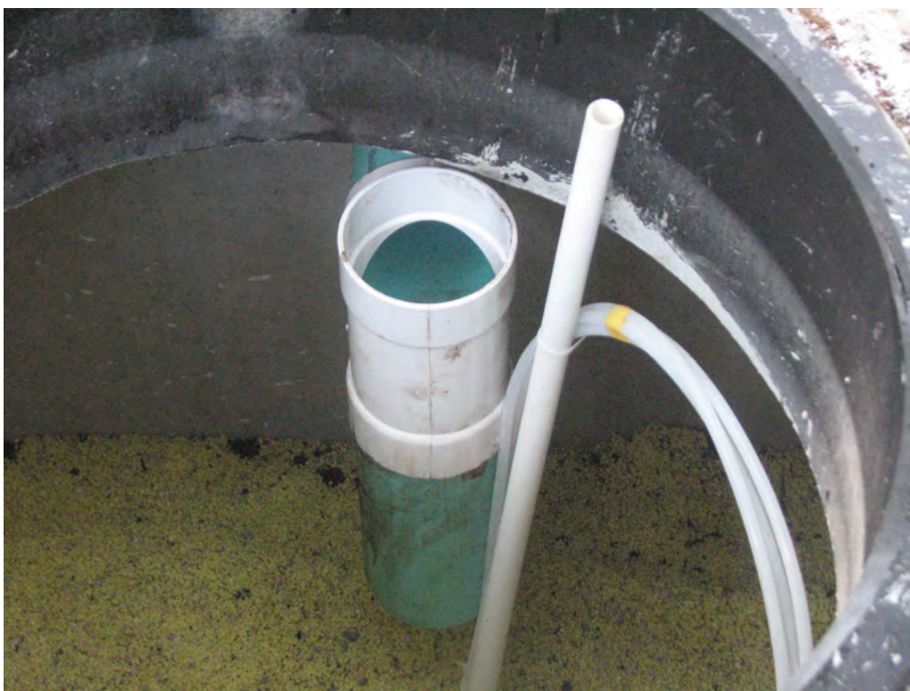
Figure 26 Stage 2 biofilter tank outlet tee
