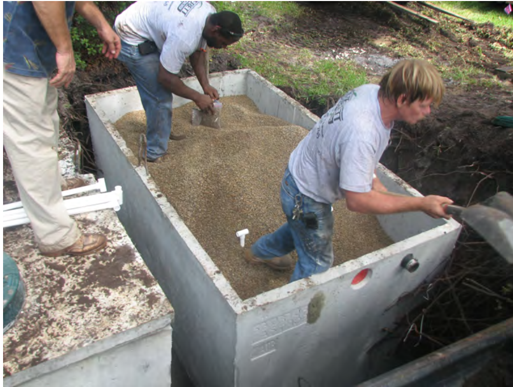
Figure 10 Stage 1 biofilter 10-inches of coarse media (1/4 Riverlite™)
