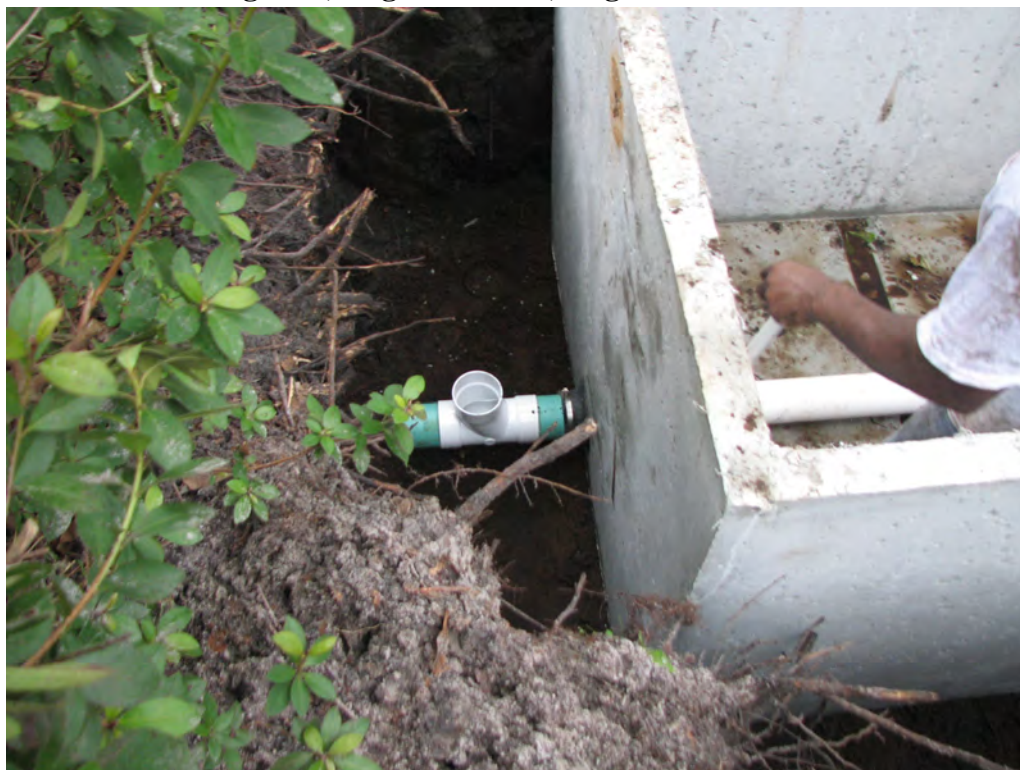
Figure 7 Stage 1 biofilter 4-inch diameter outlet pipe, with cleanout
