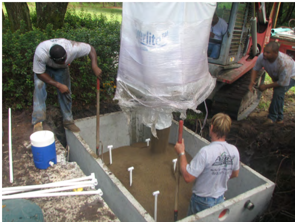
Figure 9 Stage 1 biofilter 20-inches of fine media (3/16 Riverlite™)
