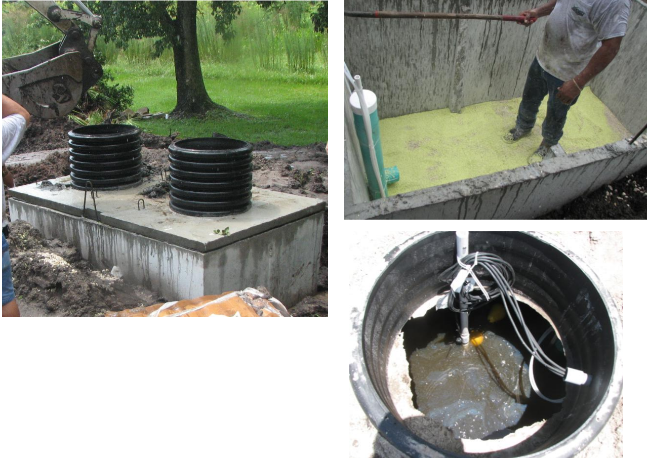
Figure 14 Stage 2 Biofilter
