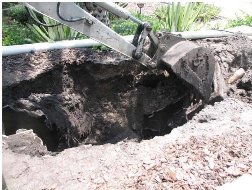
Figure 3 Old septic tank pumped out and removed
