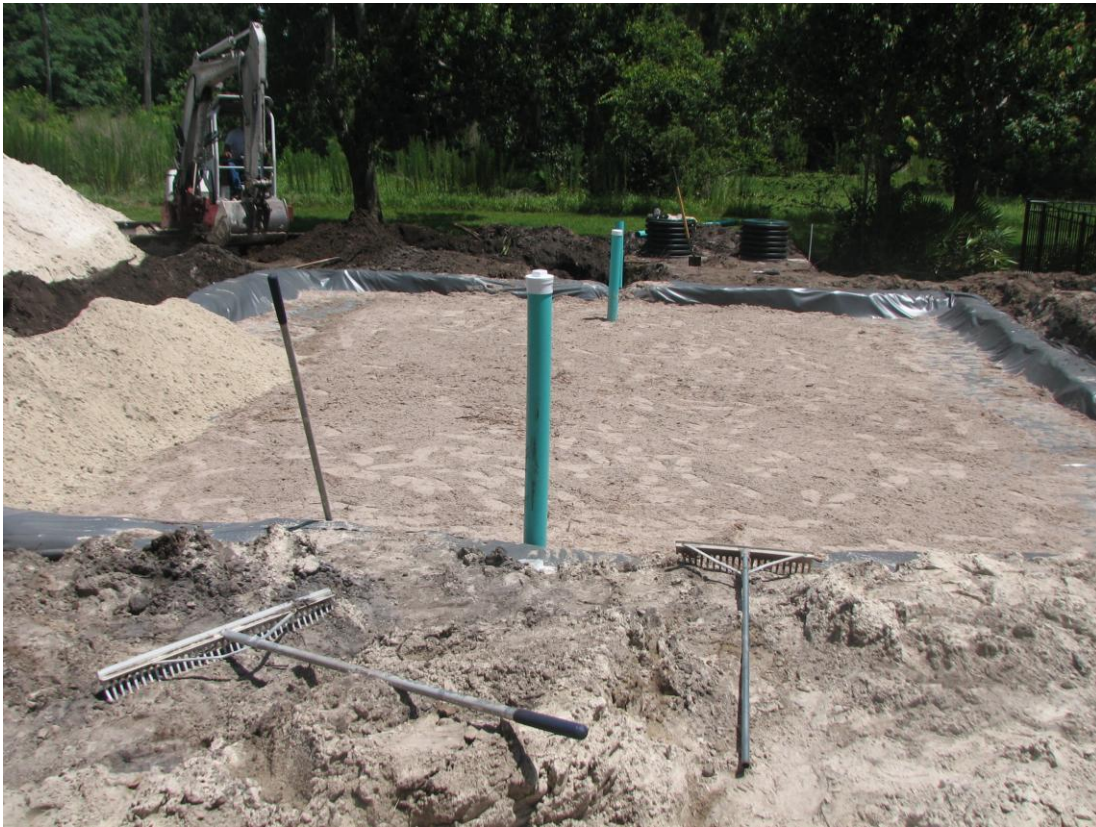
Figure 12 Lignocellulosic and sand mixture above liner
