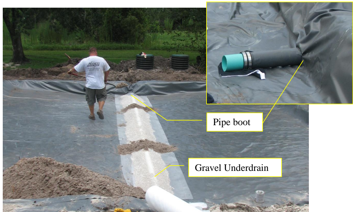
Figure 10 Stage 1 liner area preparation
