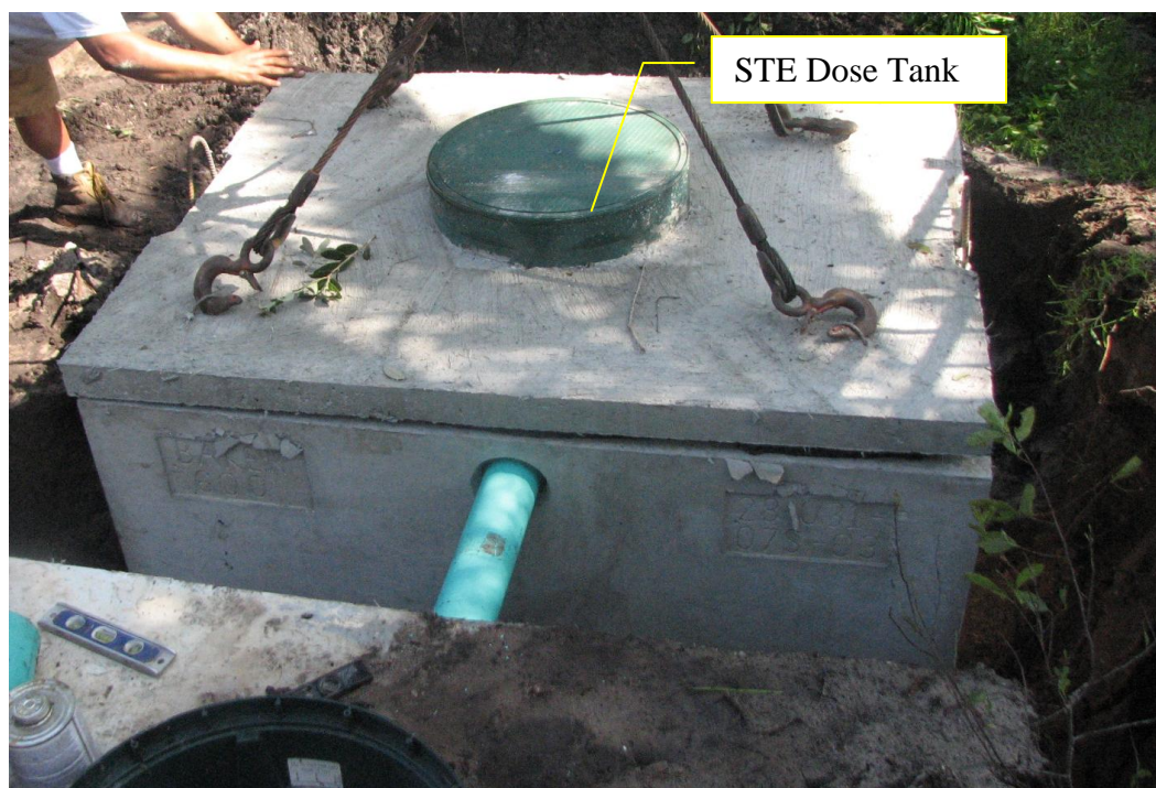
Figure 6 600 gallon, single chamber, STE Dose Tank
