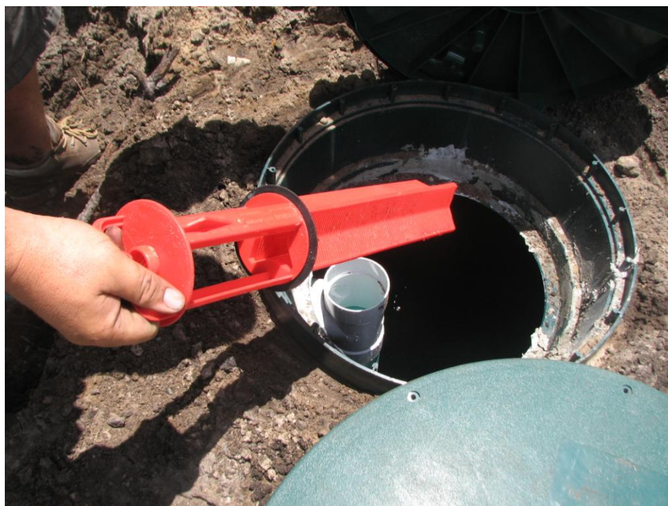
Figure 5 Primary tank effluent screen
