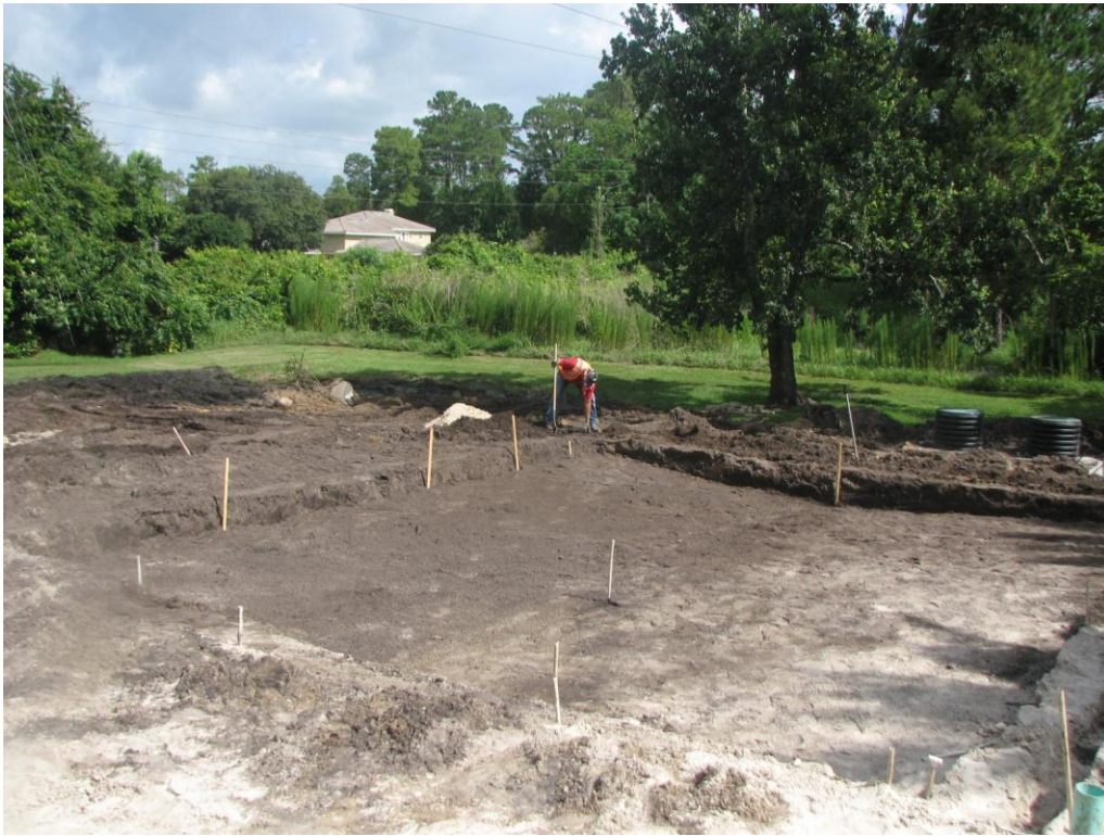
Figure 10 Stage 1 liner area preparation
