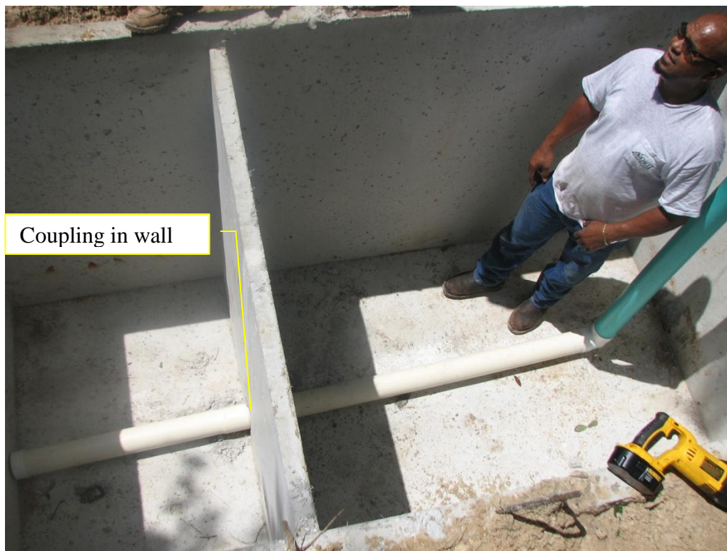
Figure 13 Stage 2 biofilter perforated pipe through wall
