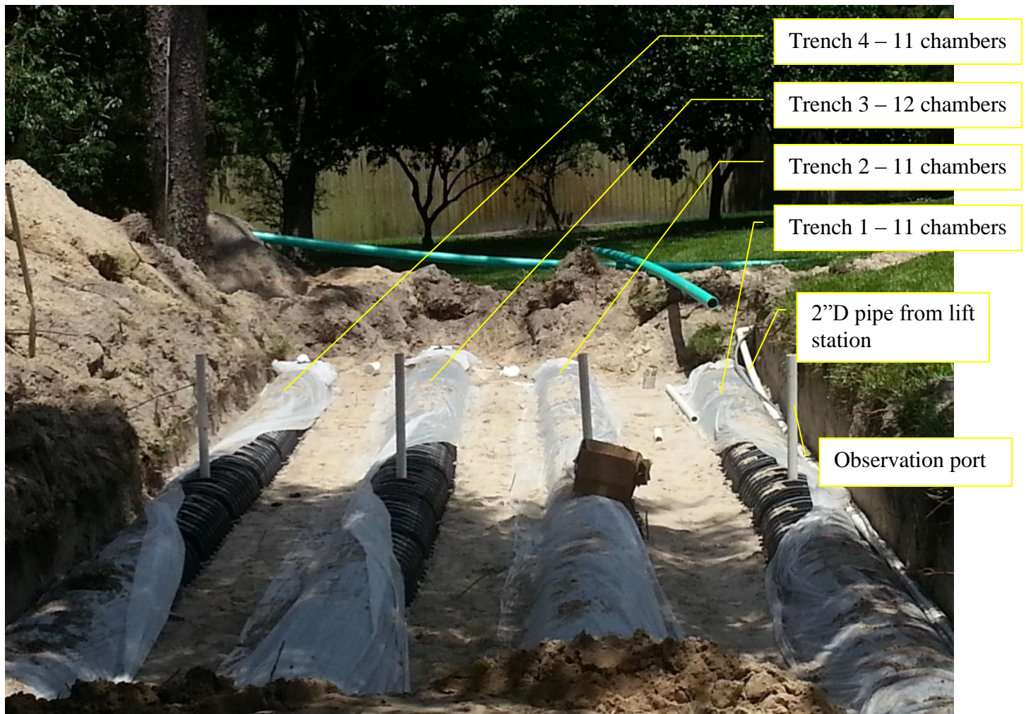
Figure 19 Drainfield trenches
