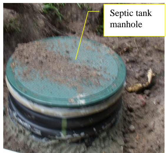
Figure 5 Septic tank outlet screen and manhole
