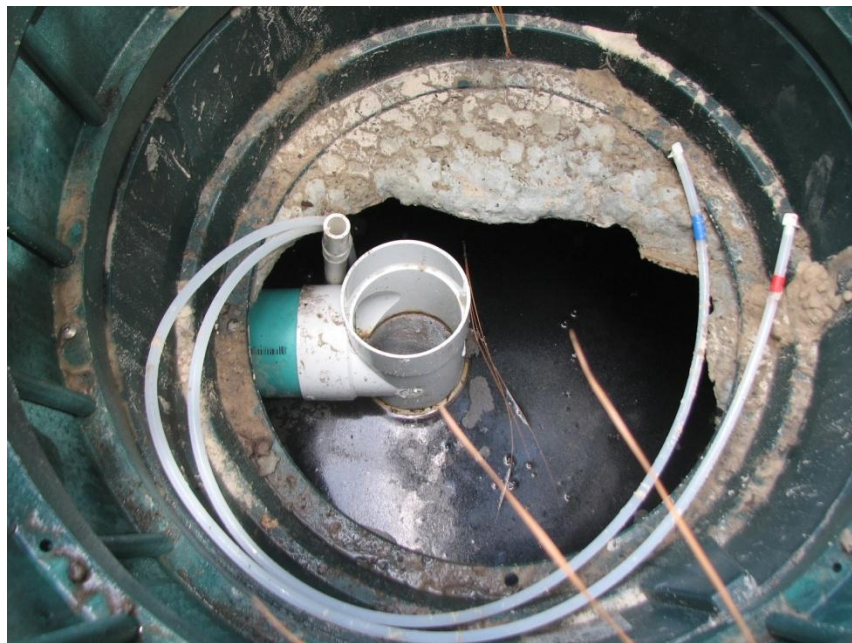
Figure 17 Stage 2 biofilter outlet tee
