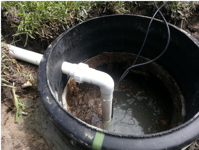
Figure 4 Liberty pump within lift station
