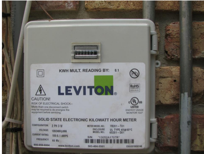
Figure 20 Power meter inside outdoor enclosure
