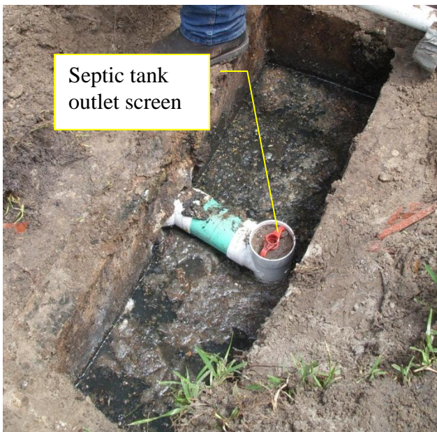
Figure 5 Septic tank outlet screen and manhole
