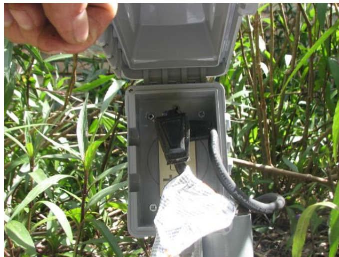
Figure 21 Power outlet for grinder pump in lift station
