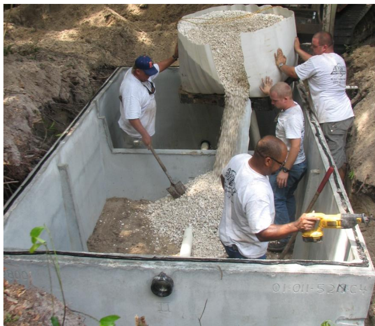
Figure 8 Stage 1 biofilter gravel underdrain
