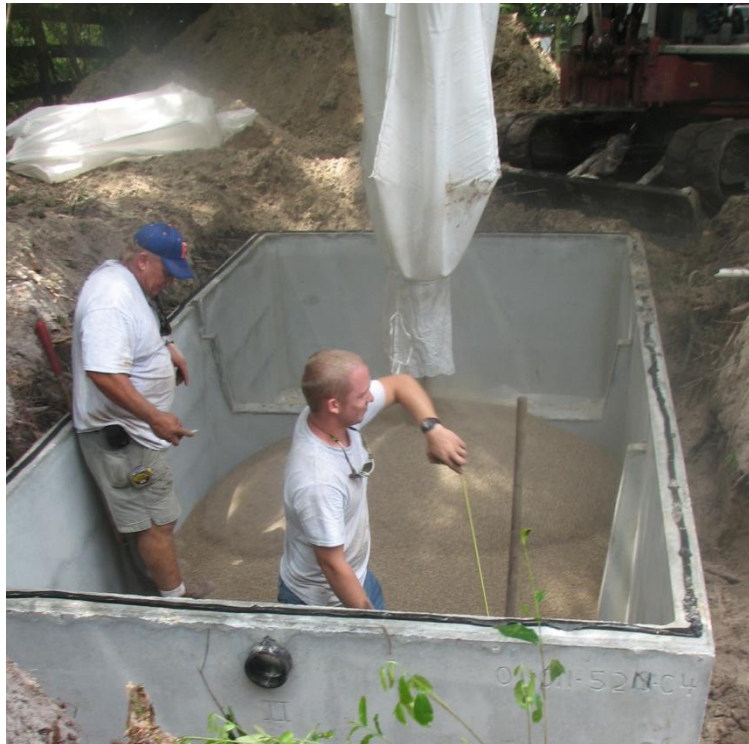
Figure 9 Stage 1 biofilter 20-inches of fine media (3/16 Riverlite™)
