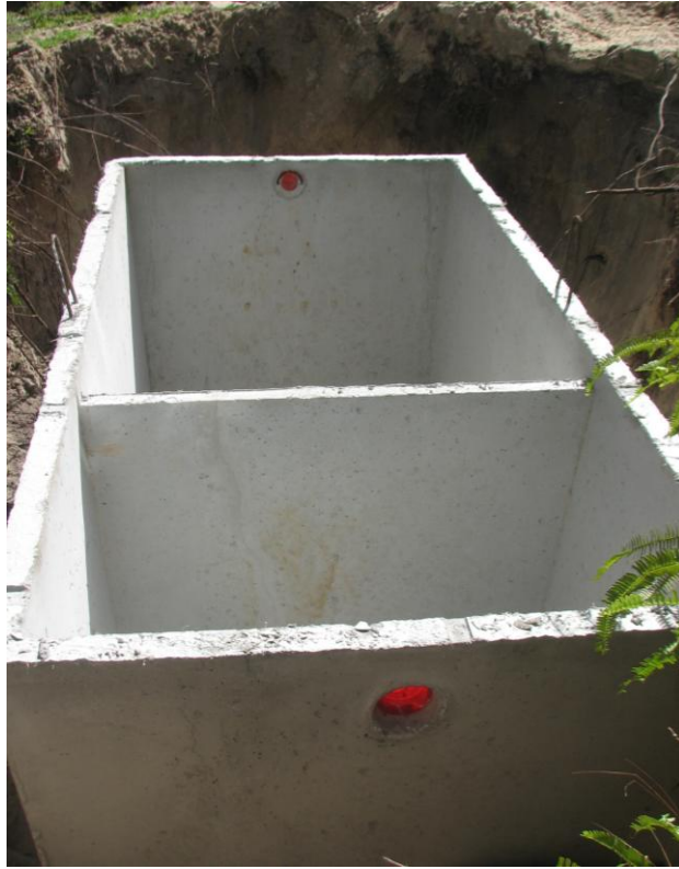
Figure 16 1,500 gallon stage 2 biofilter tank
