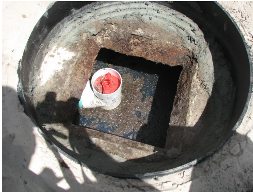
Figure 6 1,350 gallon, primary Tank effluent screen
