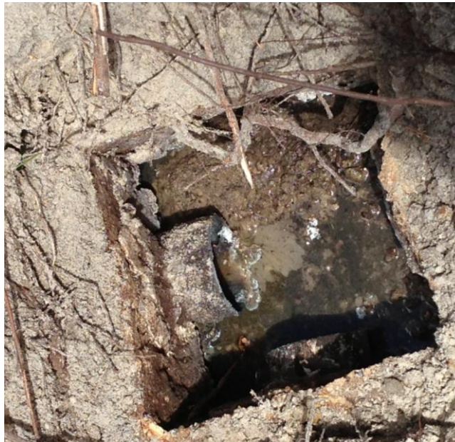
Figure 4 Existing drainfield distribution box
