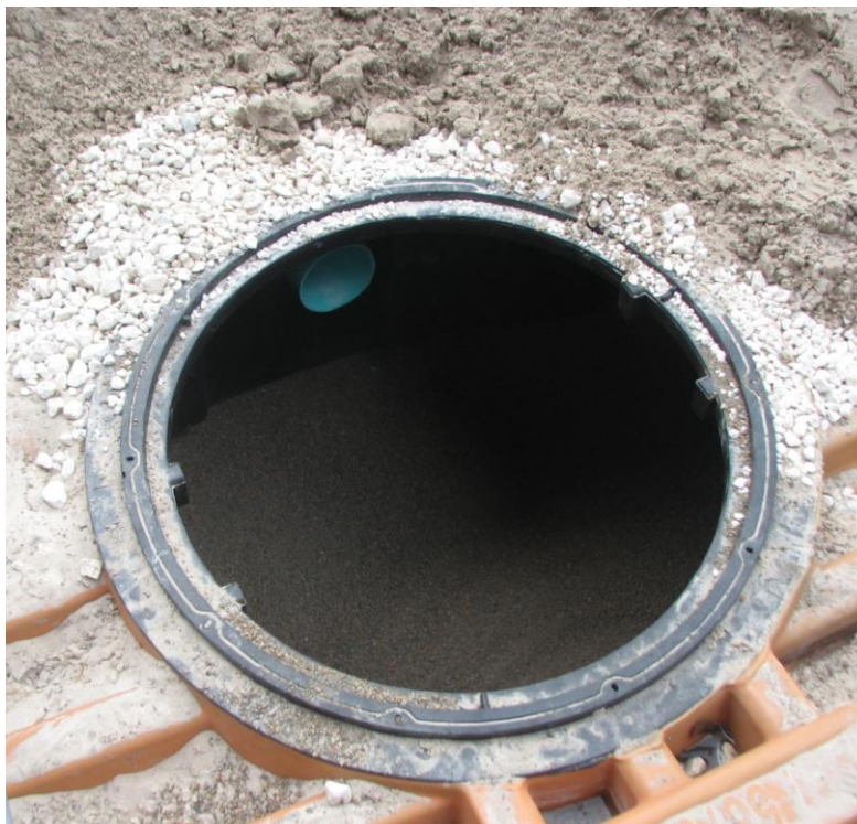
Figure 10 Stage 1 biofilter 21-inches of fine media (3/16 Riverlite™)
