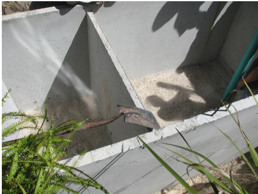
Figure 17 Stage 2 biofilter tank gravel underdrain covering perforated pipe along bottom
