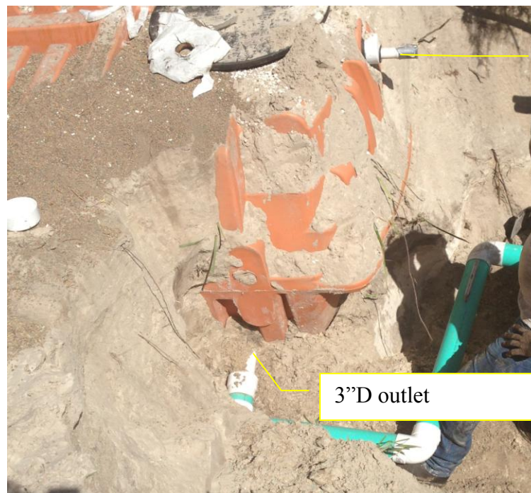
Figure 8 Stage 1 biofilter 3\"D outlet pipe, with cleanout
