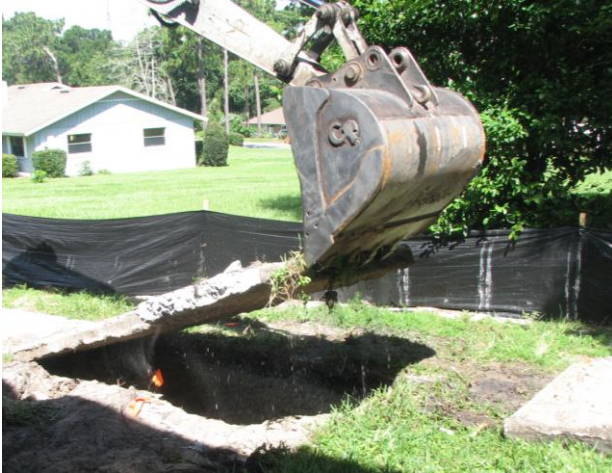
Figure 3 Concrete sidewalk removed
