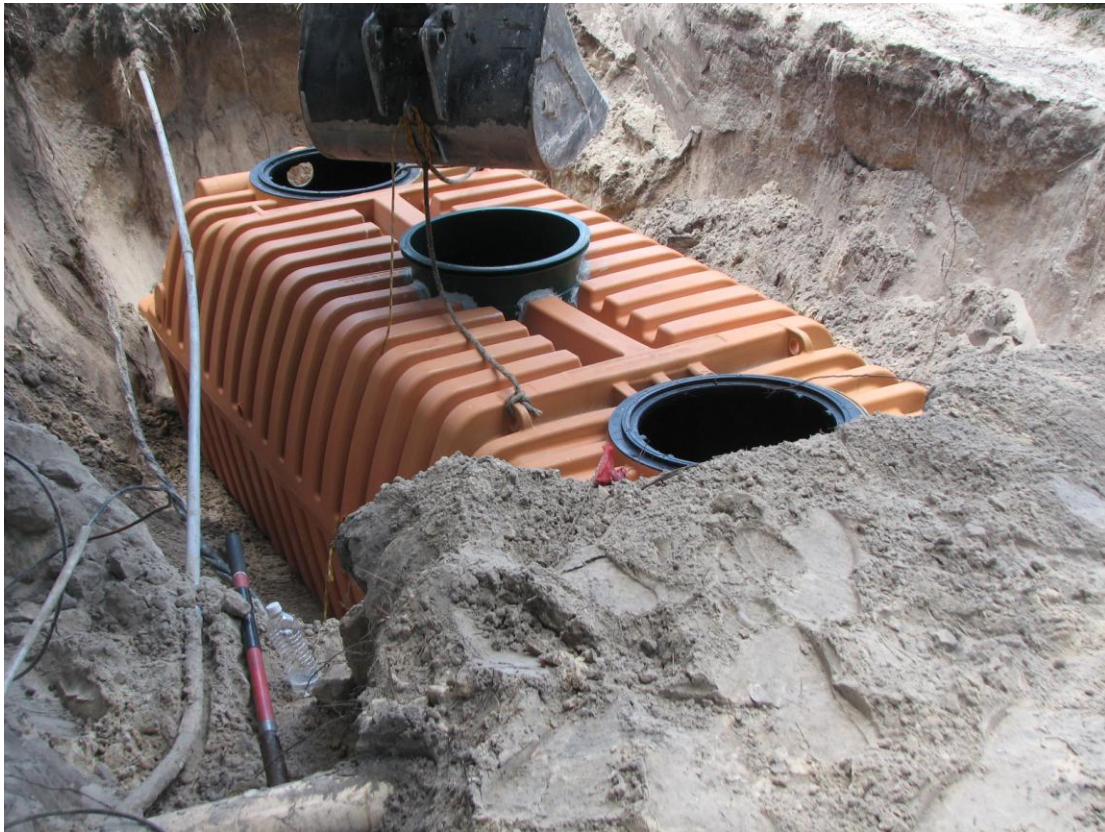
Figure 7 1500 gallon, single chamber, stage 1 biofilter tank
