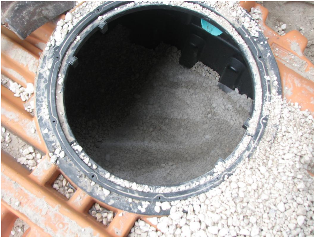
Figure 9 Stage 1 biofilter gravel underdrain
