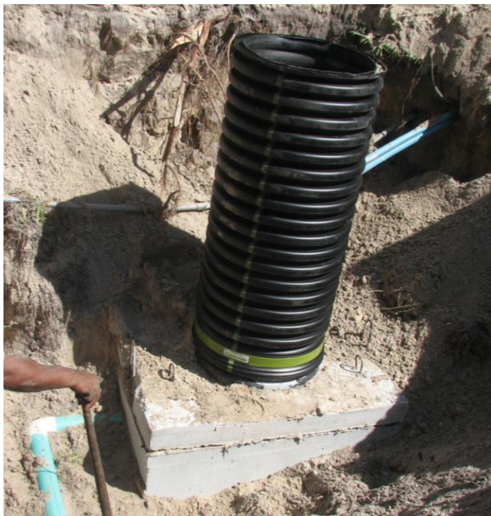
Figure 13 300 gallon pump tank
