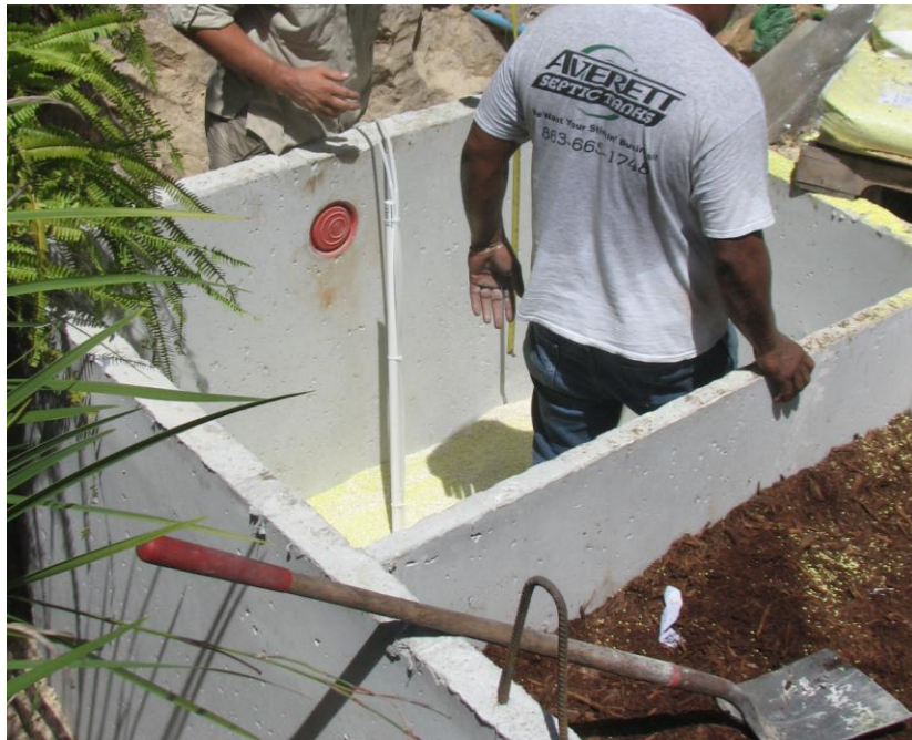
Figure 18 Stage 2 biofilter tank (sulfur mixed with oyster shell)
