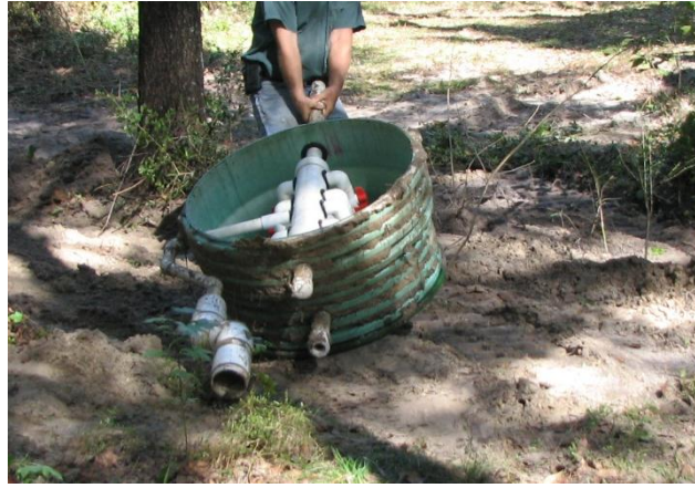
Figure 7 Split Recirculation Device removal
