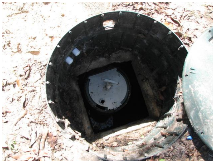
Figure 4 Primary tank effluent screen moved to outlet
