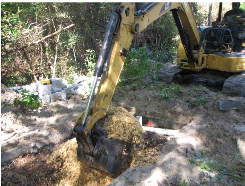
Figure 6 Nitrex™ media removal
