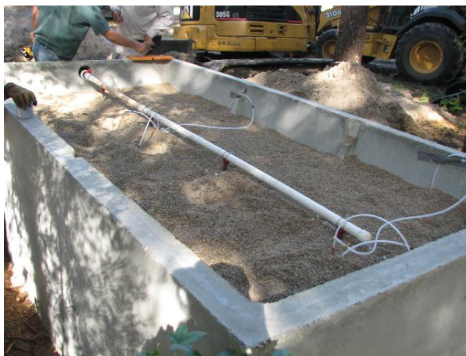
Figure 13 Expanded clay media installation
