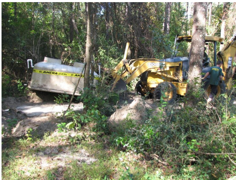
Figure 5 Aerocell™ unsaturated media filter chamber removal
