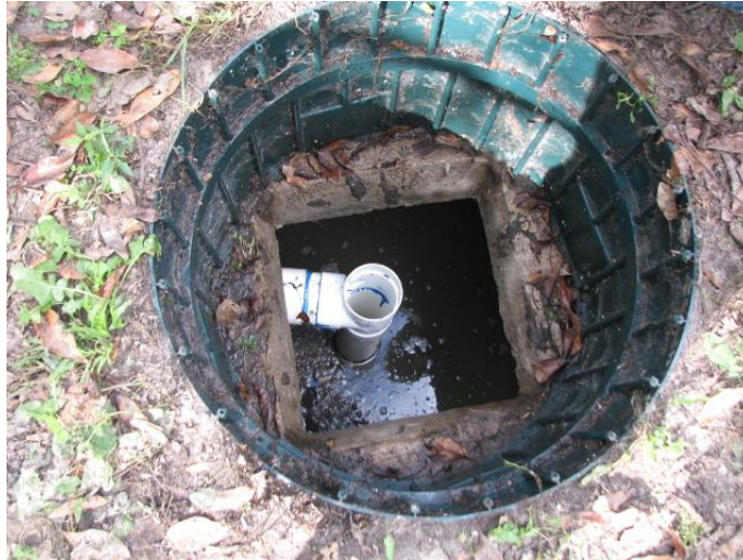
Figure 3 Primary tank vented tee between chambers
