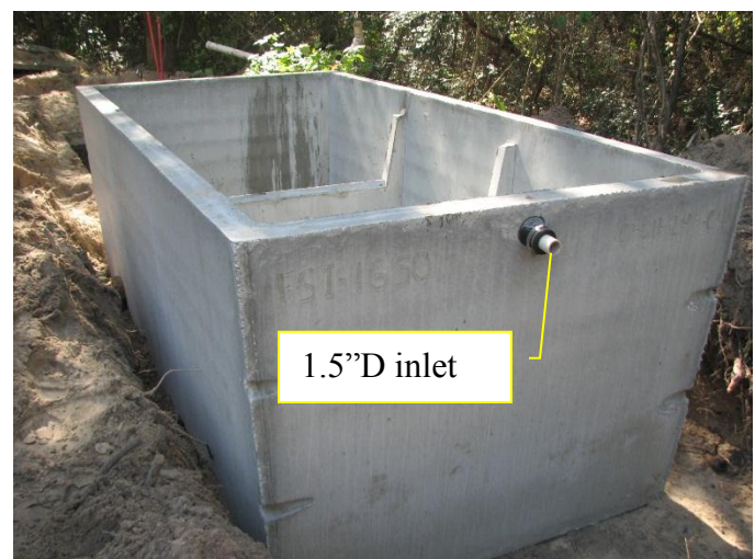
Figure 11 Combination Stage 1 and 2a Biofilter (1650 gallon)
