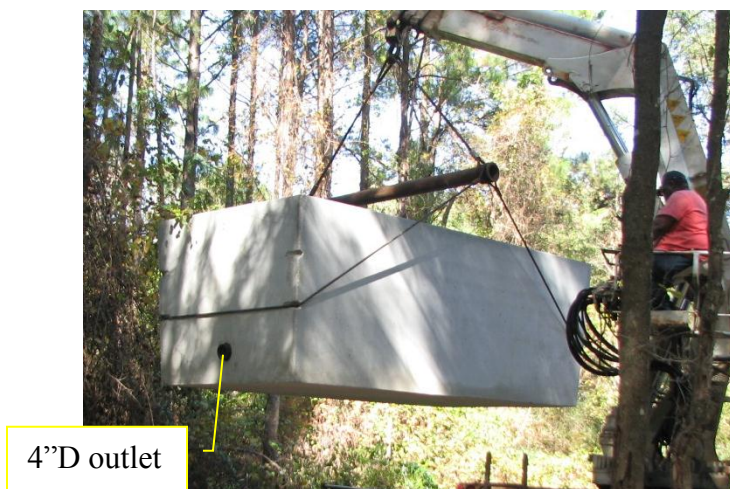
Figure 11 Combination Stage 1 and 2a Biofilter (1650 gallon)
