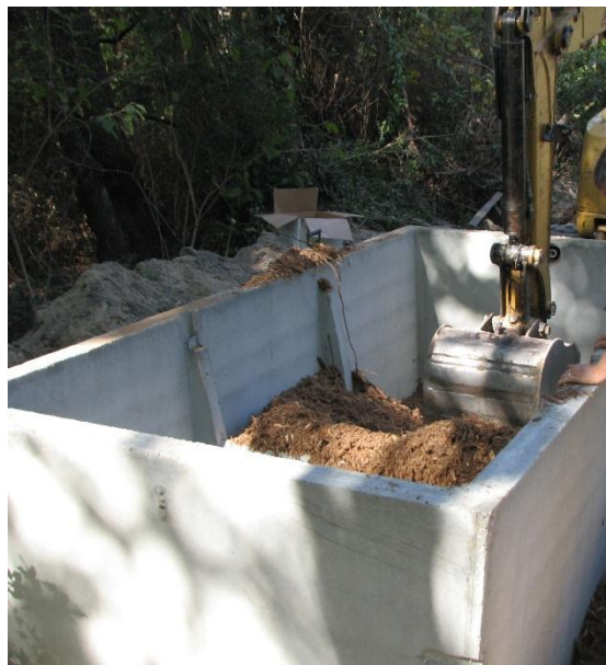
Figure 12 Lignocellulosic media installation
