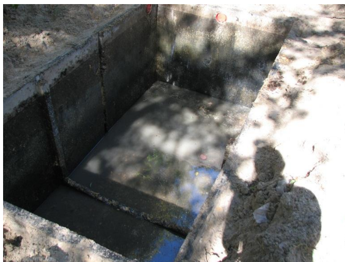
Figure 17 Cleaned Stage 2b tank (1500 gallon)
