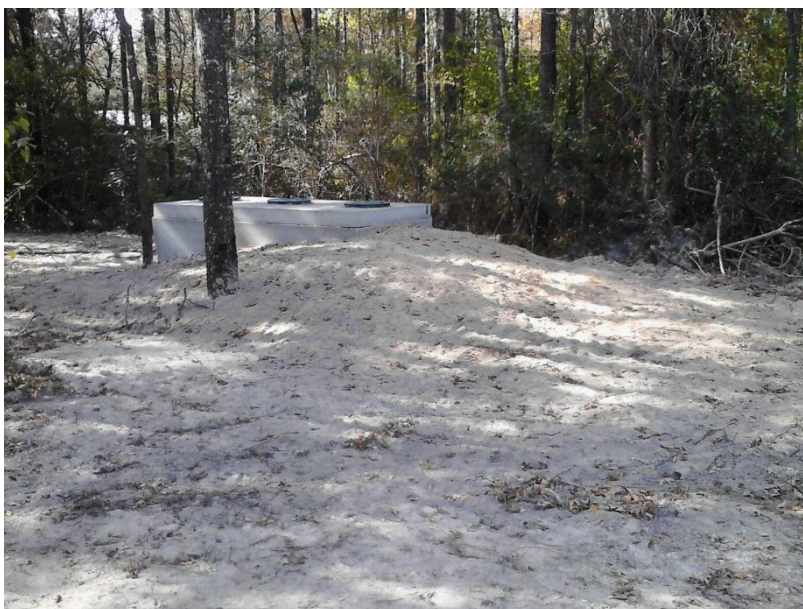
Figure 16 Stage 1 and Stage 2a berm hiding tank
