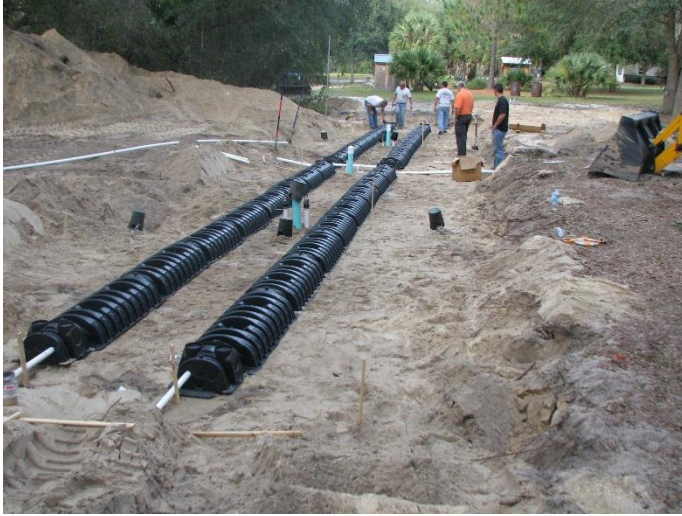
Figure 15 Infiltrator chambers
