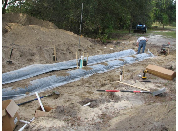
Figure 15 Infiltrator chambers
