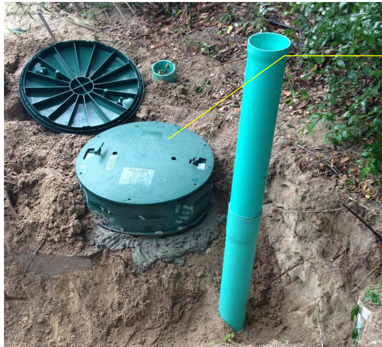
Figure 3 Primary tank access riser and cover
