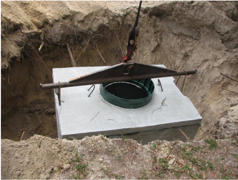
Figure 5 Pump tank (300 gallon)
