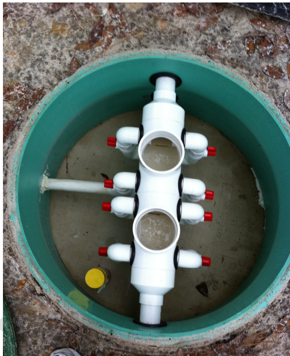
Figure 2 Photo of Split Recirculation Device installed December 9, 2011
