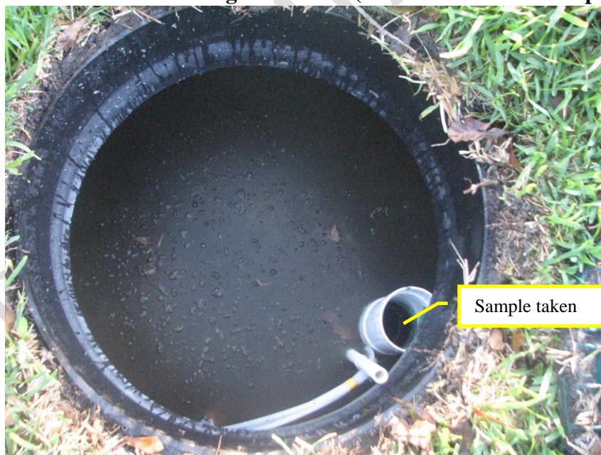
Figure 7 First chamber of Stage 2 biofilter (B-HS2-LIGNO-0" sample)
