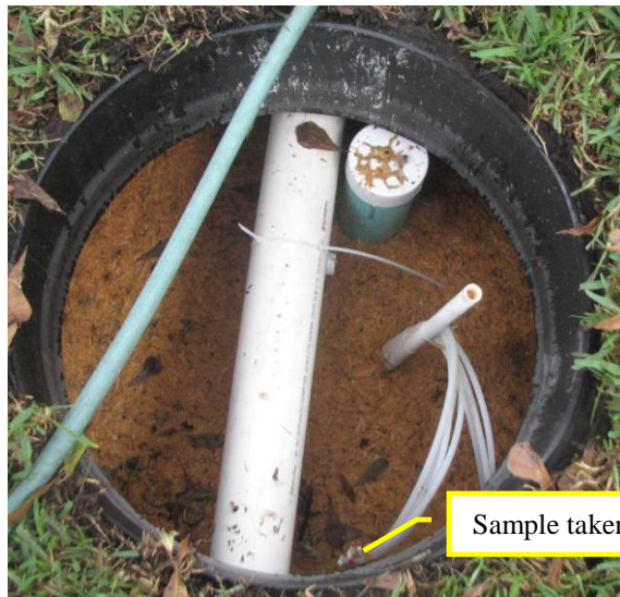
Figure 7 First chamber of Stage 2 biofilter (B-HS2-LIGNO-0" sample)
