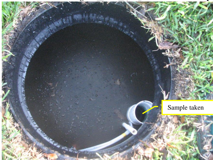
Figure 7 First chamber of Stage 2 biofilter (B-HS2-LIGNO-0" sample)
