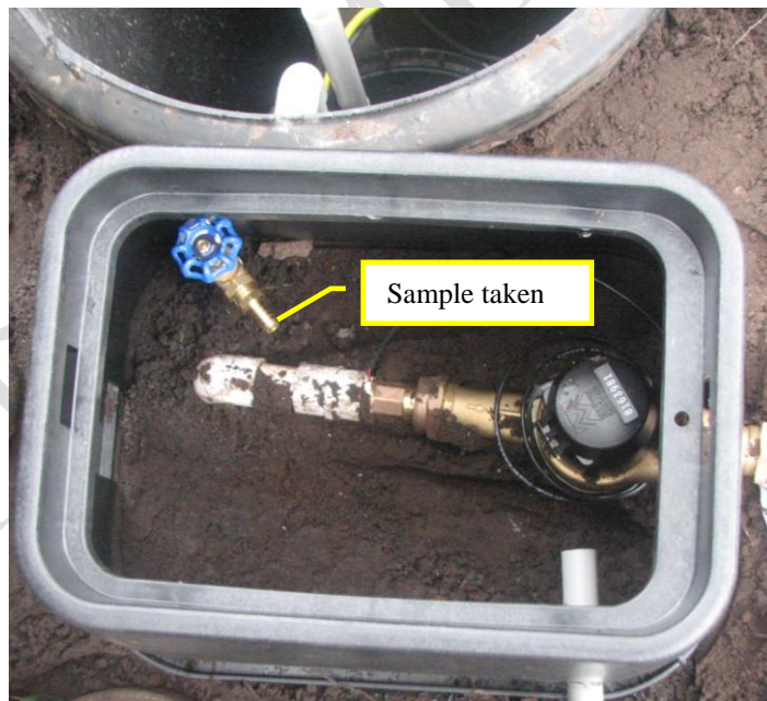
Figure 6 Pump discharge line sample port (B-HS2-PUMP sample)
