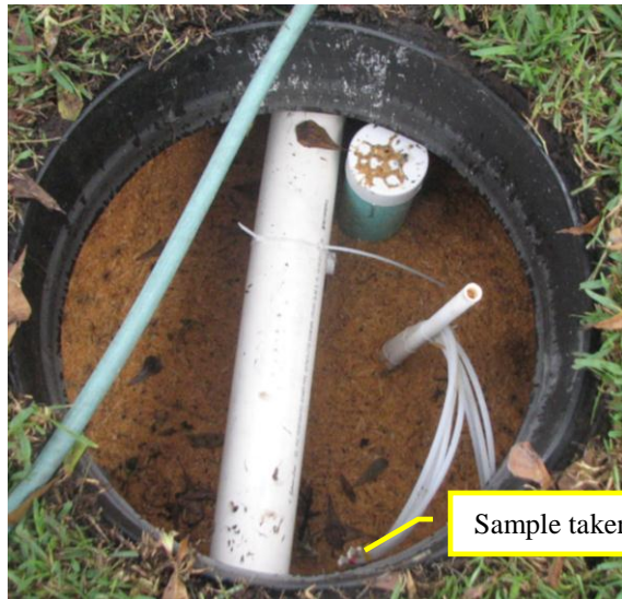
Figure 6 First chamber of Stage 2 biofilter (B-HS2-LIGNO-0 sample)
