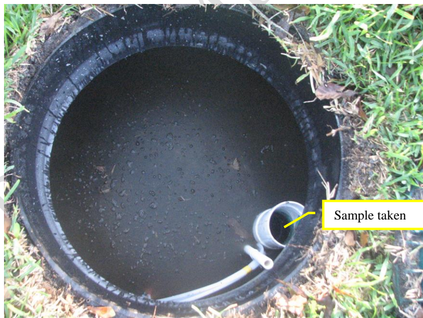
Figure 7 Second Chamber of Stage 2 Biofilter (B-HS2-ST2 Sample)
