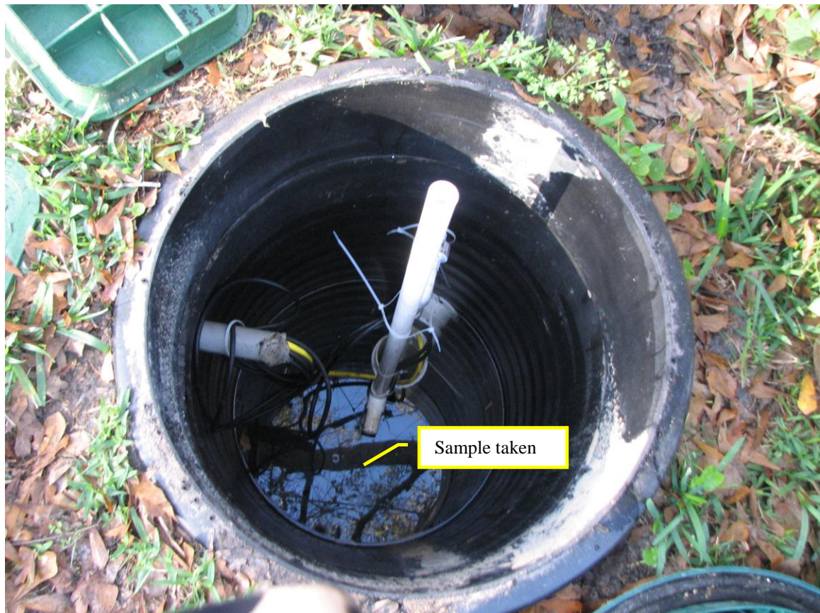
Figure 5 Stage 1 effluent sample taken in pump tank (B-HS2-ST1 sample)
