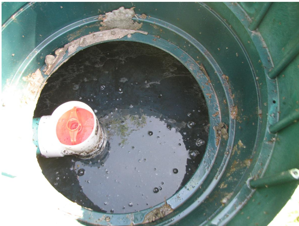
Figure 5 Second Chamber of Primary Tank (B-HS3-STE Sample)
