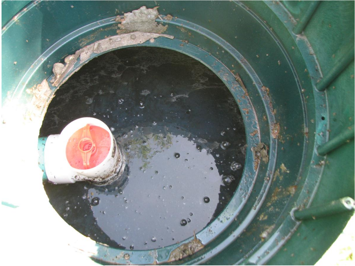
Figure 4 Second Chamber of Primary Tank (B-HS3-STE Sample)
