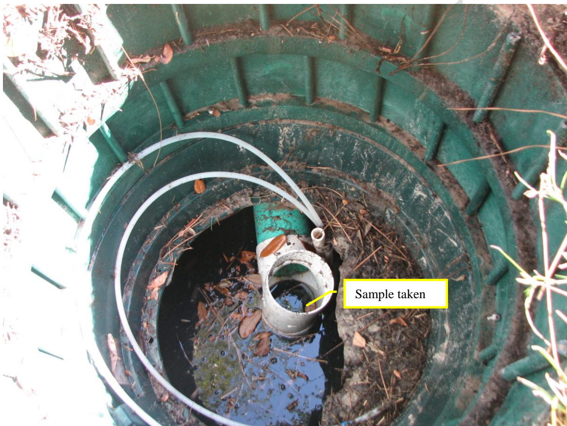
Figure 6 Second chamber of Stage 2 biofilter (B-HS4-ST2 sample)
