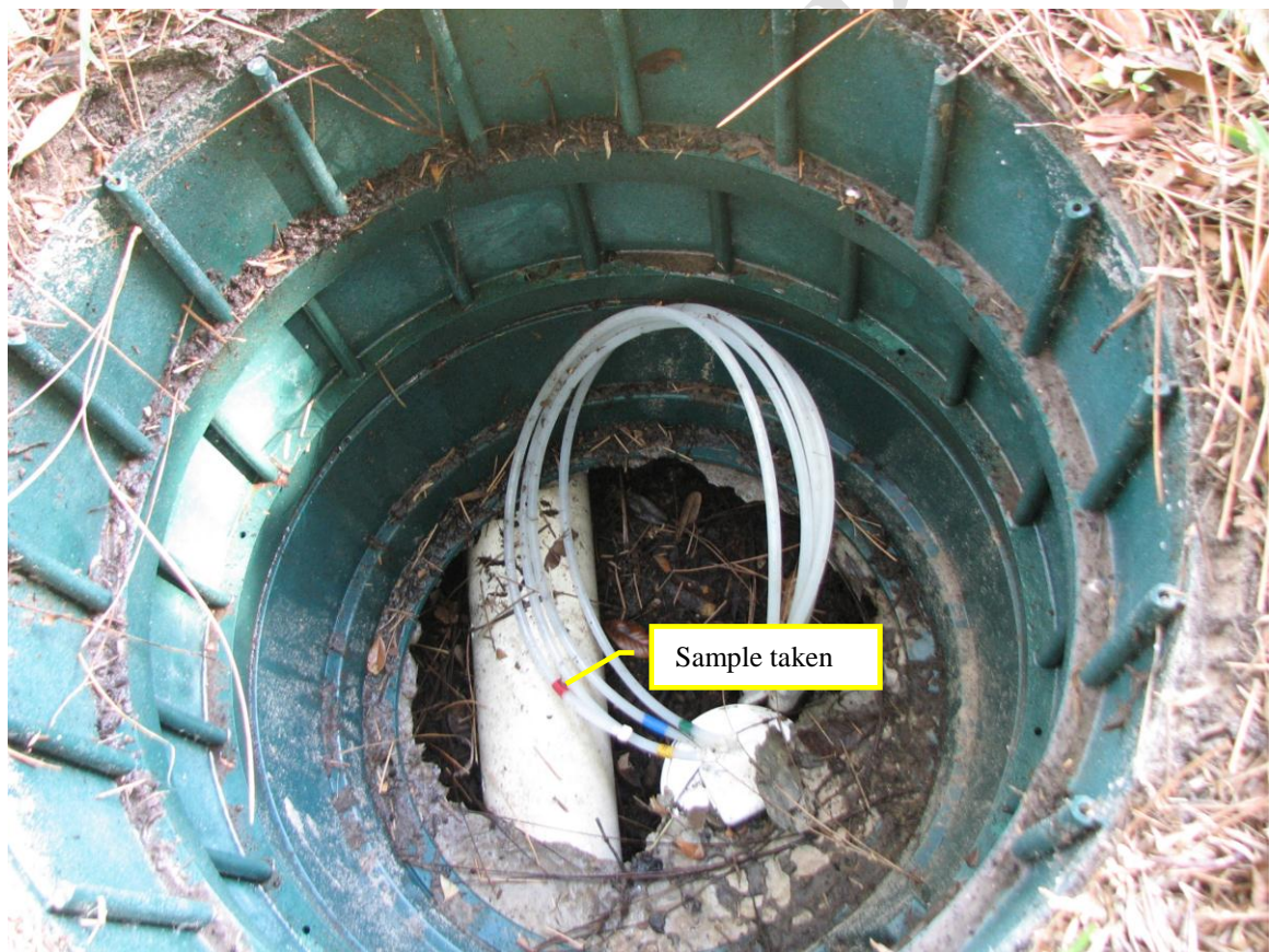
Figure 5 First chamber of Stage 2 biofilter (B-HS4-LIGNO-0" sample)
