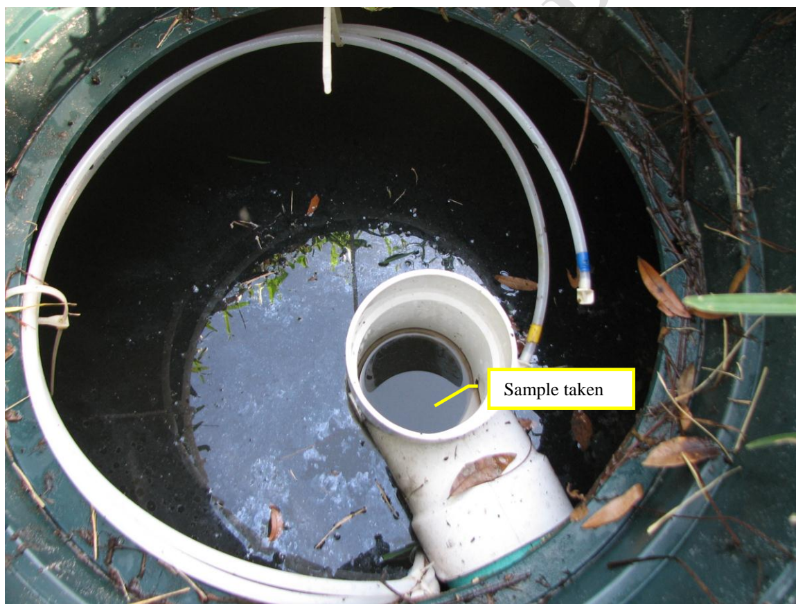
Figure 7 Second chamber of Stage 2 biofilter (B-HS5-ST2 sample)
