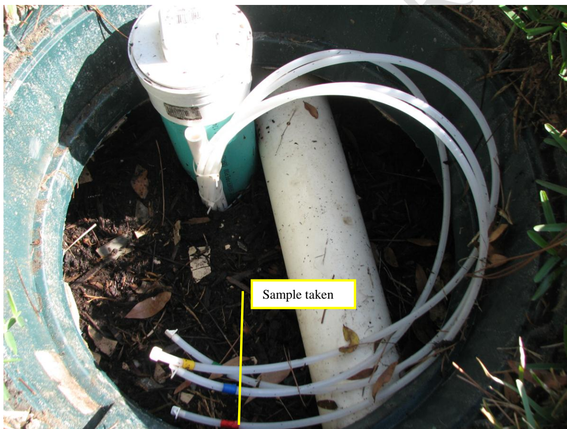
Figure 6 First chamber of Stage 2 biofilter (B-HS5-LIGNO-0" sample)
