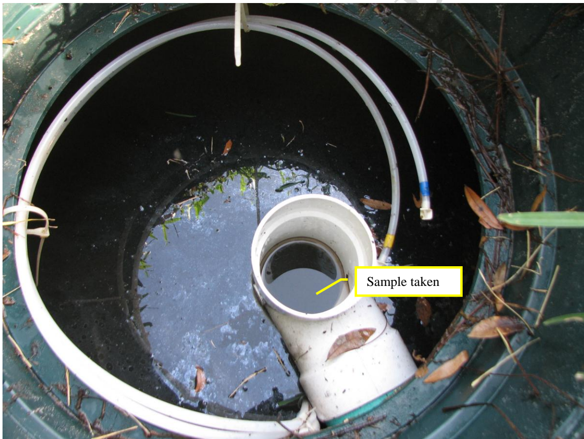
Figure 7 Second chamber of Stage 2 biofilter (B-HS5-ST2 sample)
