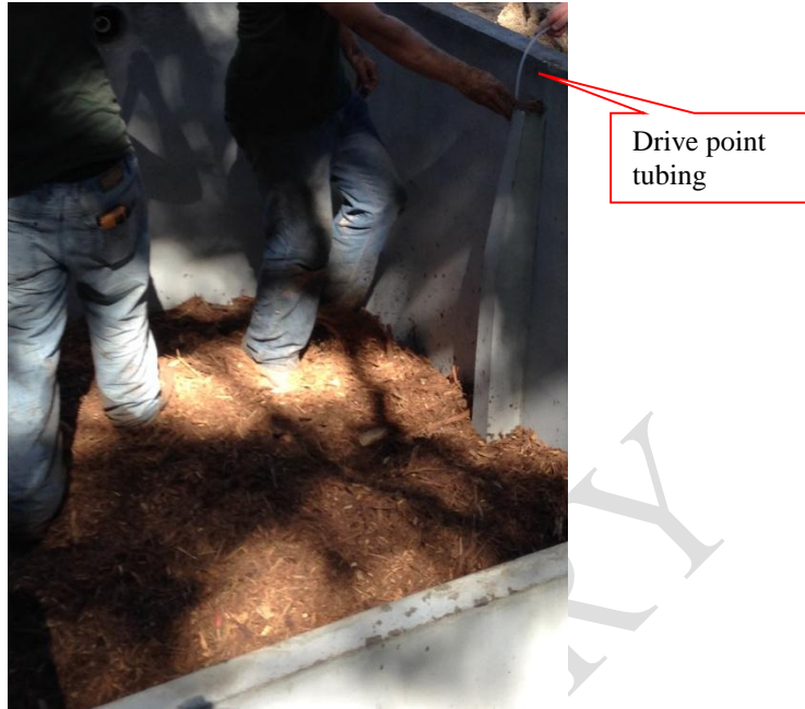
Figure 6 Stage 2a Saturated Biofilter Effluent (B-HS6-DP3 and B-HS6-DP4) sample tubing
