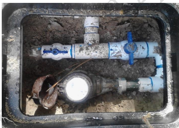
Figure 11 Treatment system flow meter
