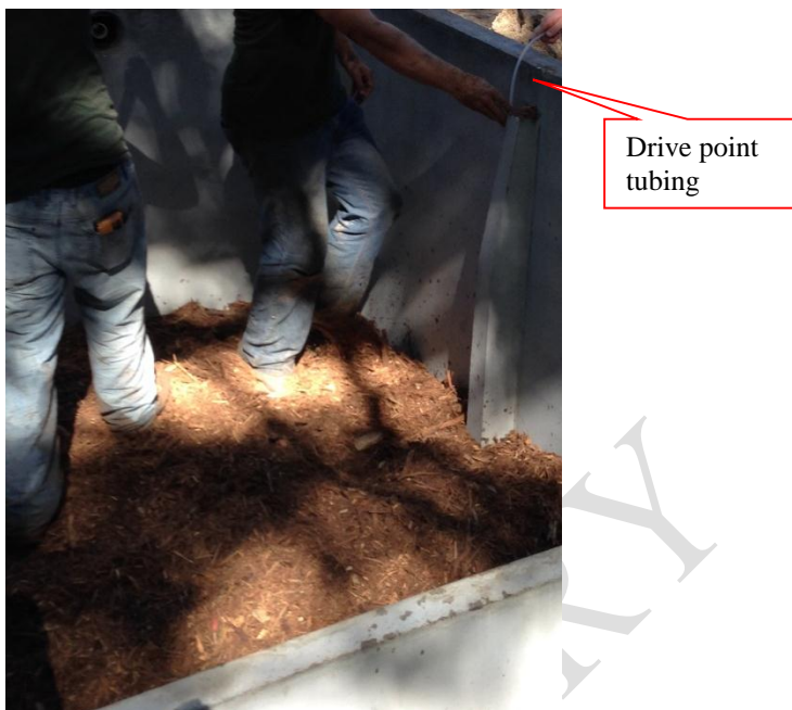
Figure 6 Stage 2a Saturated Biofilter Effluent (B-HS6-DP3 and B-HS6-DP4) sample tubing
