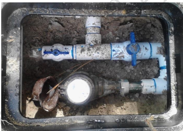
Figure 11 Treatment system flow meter
