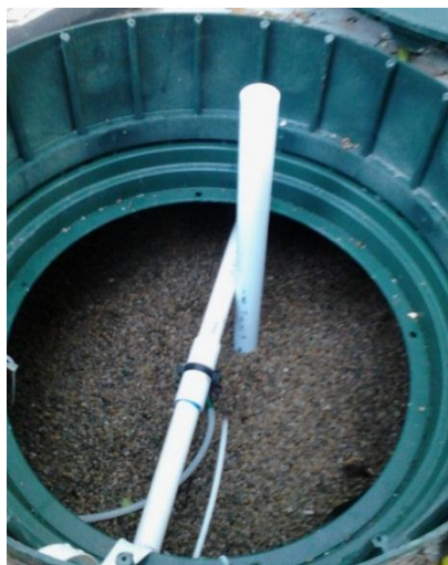
Figure 12 Piezometer installed on April 19, 2014 in the Stage 1&2a Tank
